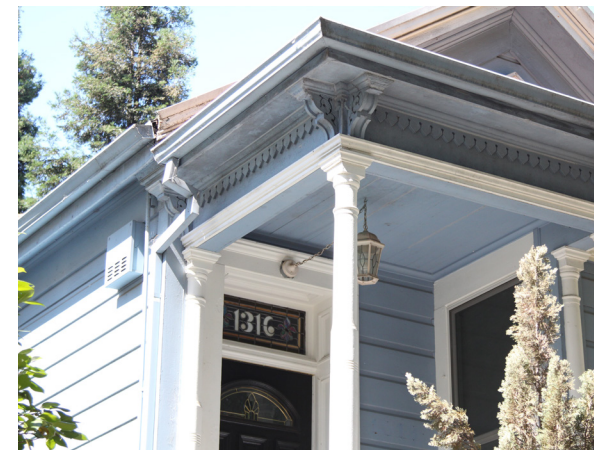
Figure 4. Decorative wood detailing and stained glass transom at a historic house in the district.
