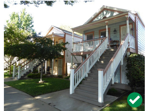
Figure 7. The replaced staircases and porch railings of these houses are compatible with the historic character of the houses and the wider historic district.
