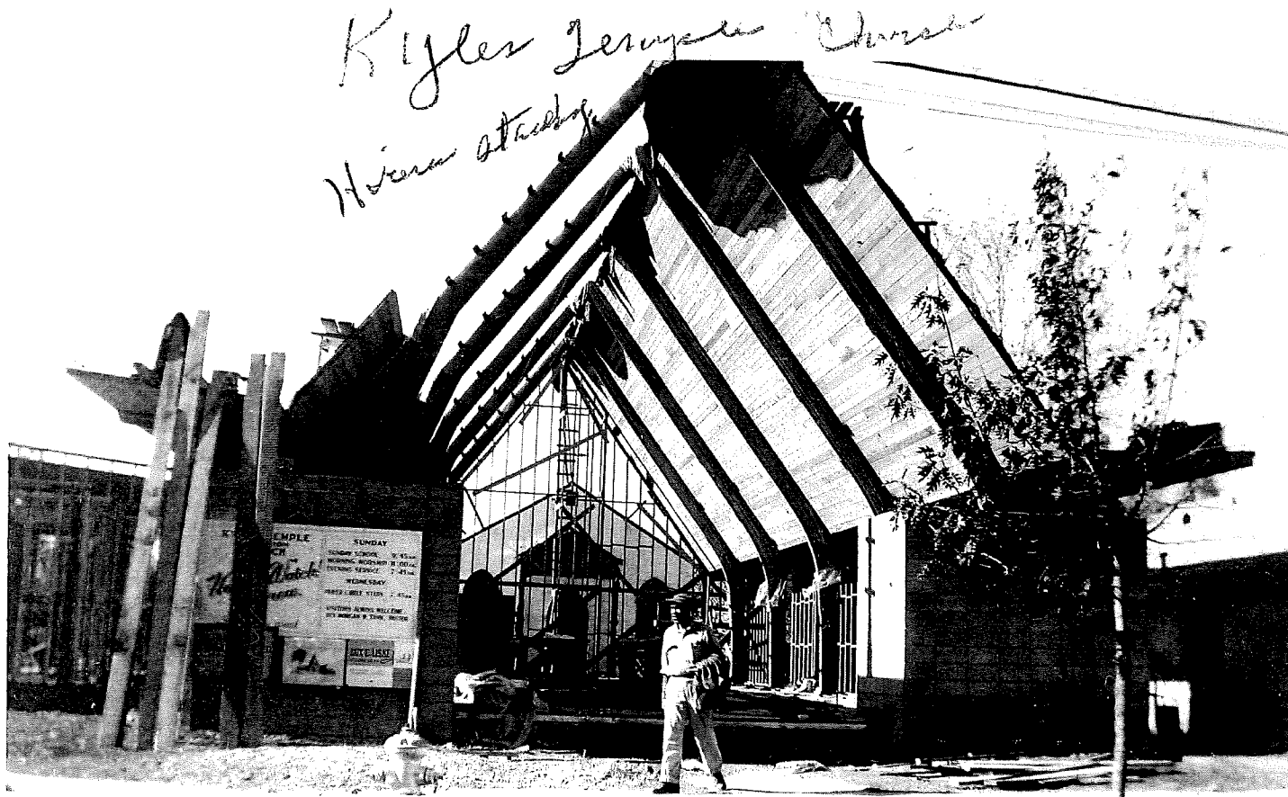
Figure 1: This photo was taken during church construction.
