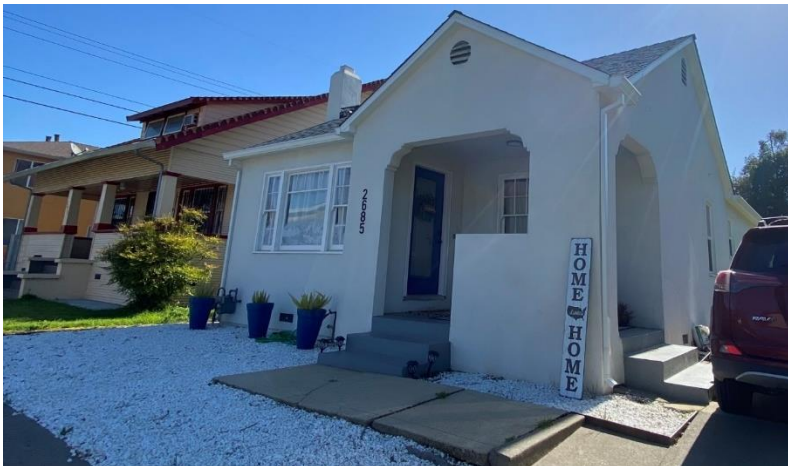
Photograph 2: Photo of west and south sides of building. Camera facing northeast.
