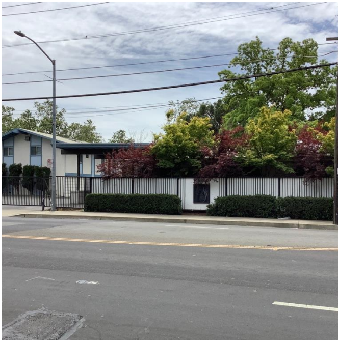
View of north facing façade, one story structures with private patio protected by privacy wall. Porte Cochere is visible at the left.
