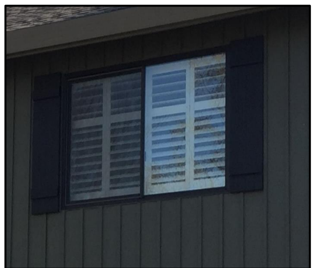
Detail of the windows.
