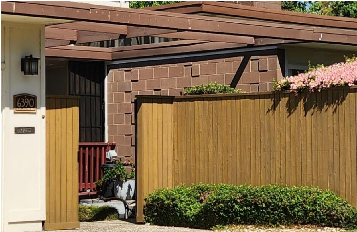
Photograph 2: Front Façade, Entry Courtyard, Camera facing northwest.
