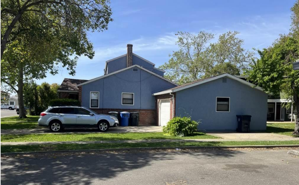
Photograph 2: North end of the house.
