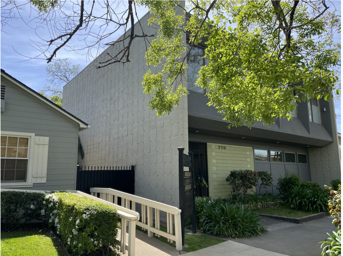
Figure 1: Photograph 2: Camera facing southwest depicting front and east facade, April 23, 2023.
