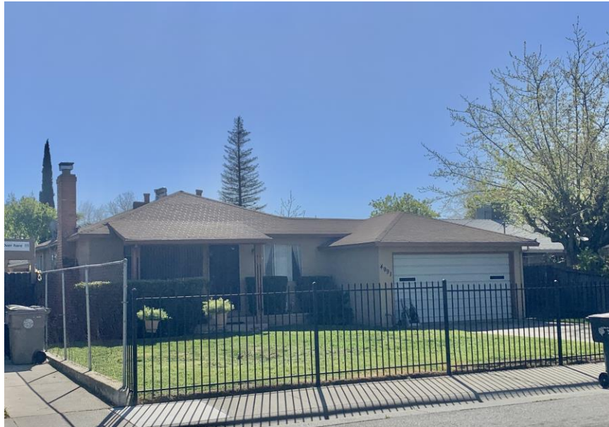
Photograph 3: 4991 Warwick Avenue, Camera facing southeast, April 13, 2023.
