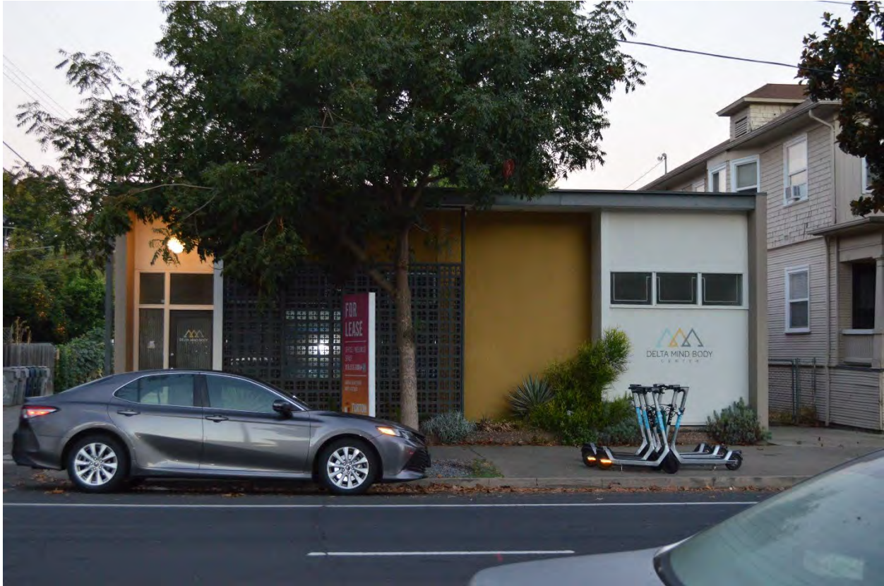
View: Front of building Facing East
