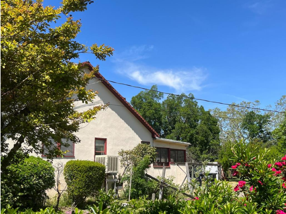
Photograph 2: East side of building, note wooden frame sash windows and covered porch at rear of home.
