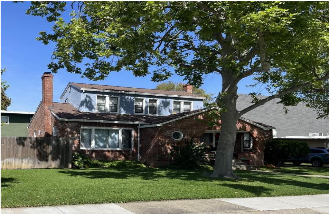
Photograph 1: Angled view of the front façade from the street.
