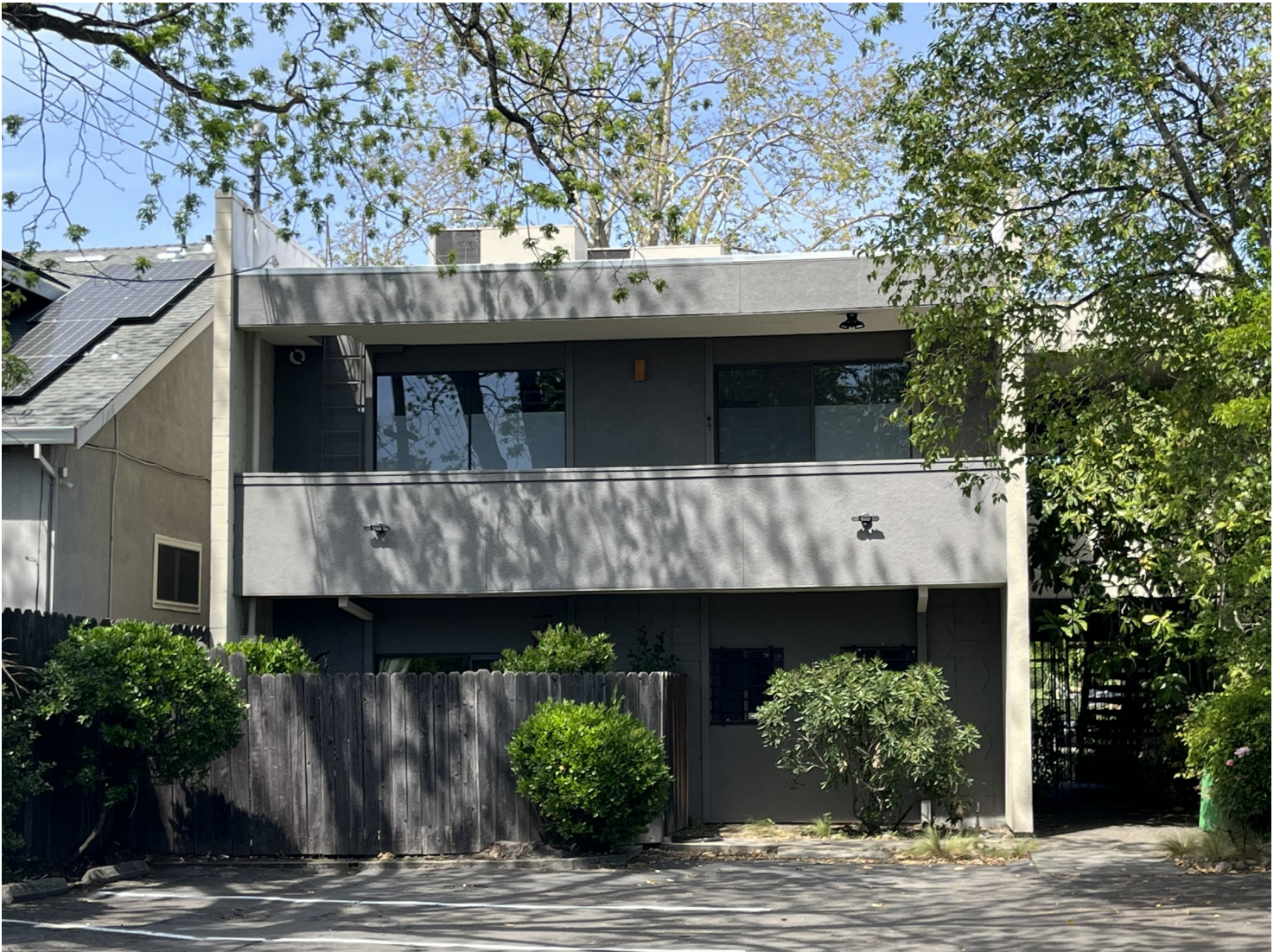
Figure 3: Photograph 4: Camera facing north depicting rear facade, April 23, 2023.
