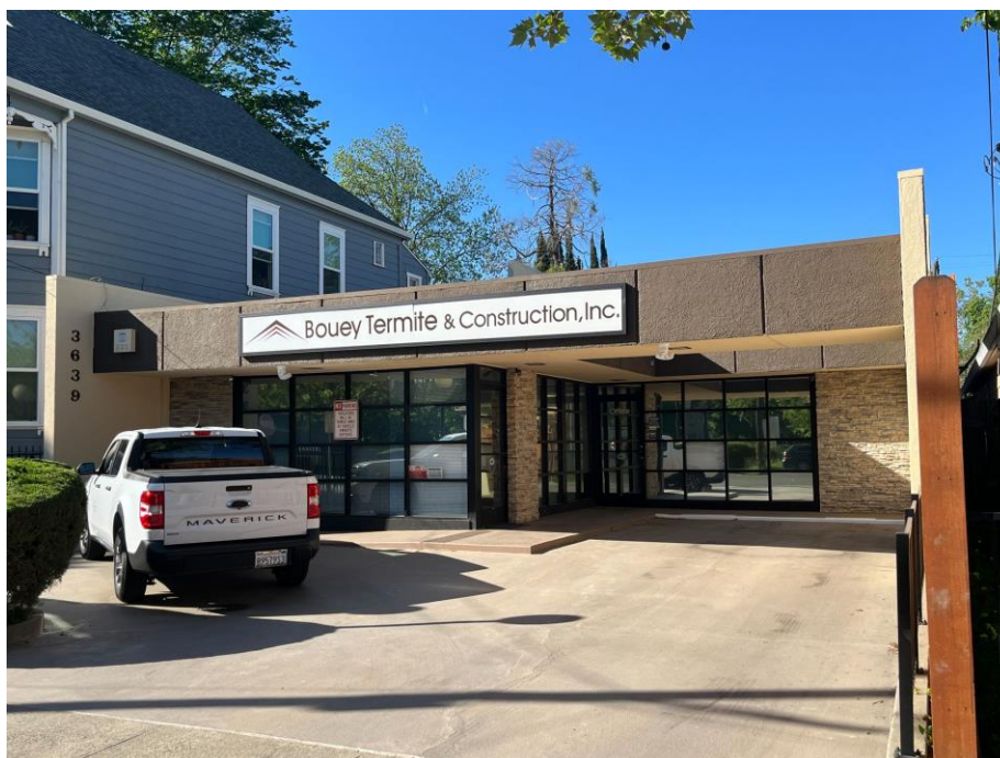
Photograph 2: Bouey Termite and Construction, Inc., facing northwest, March 27, 2023.
