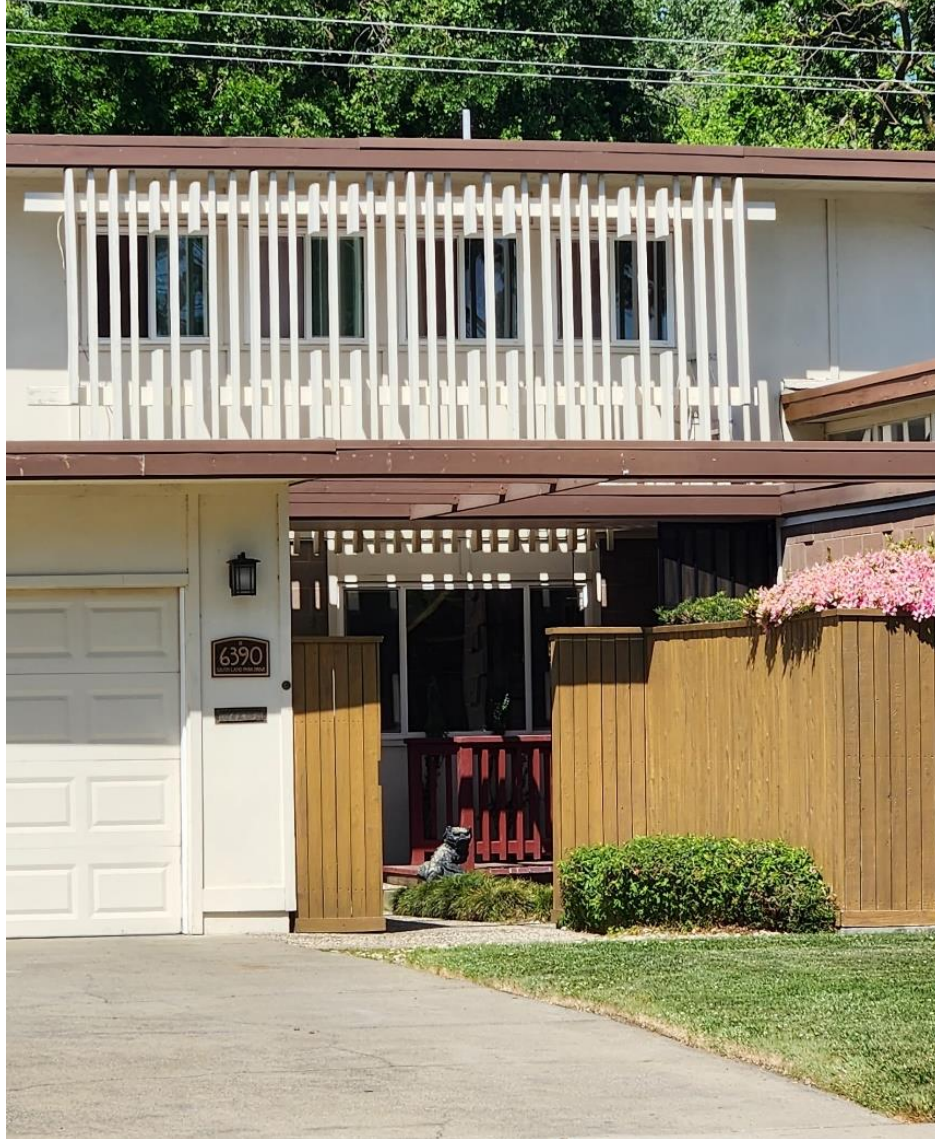
Photograph 4: Front Façade, detail shot of entry courtyard and second-floor wooden slate exterior window screen. Camera facing west
