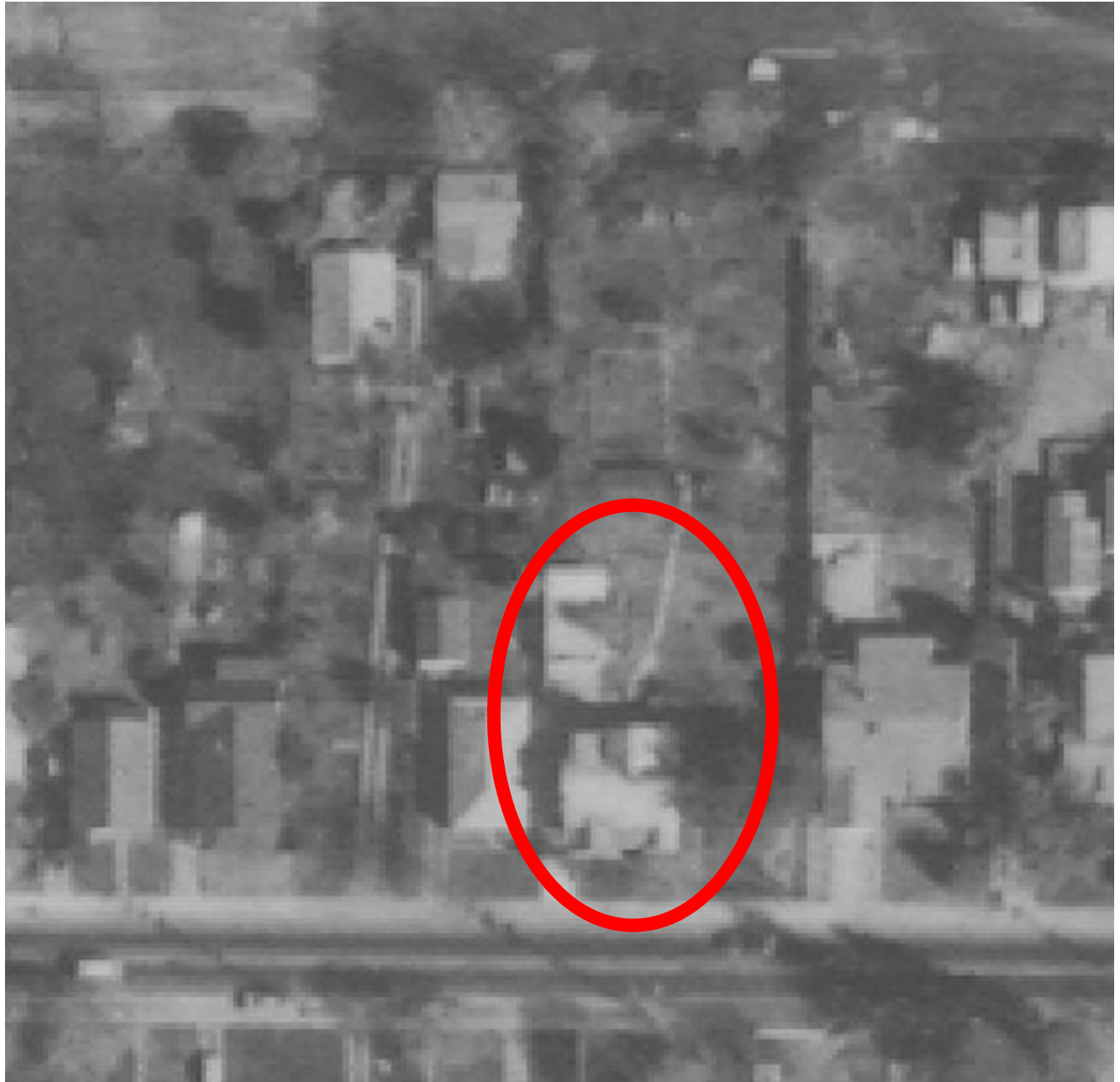
Figure 3: 1971 Aerial view of the Cooke House. Photo taken on March 1, 1971 by Cartwright Aerial Surveys. Housed at the California State Library. Note: 1971 garage appears to be identical to the extant garage.
