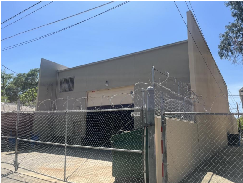
Photograph 3: Bouey Termite and Construction, Inc., facing southeast, March 27, 2023.
