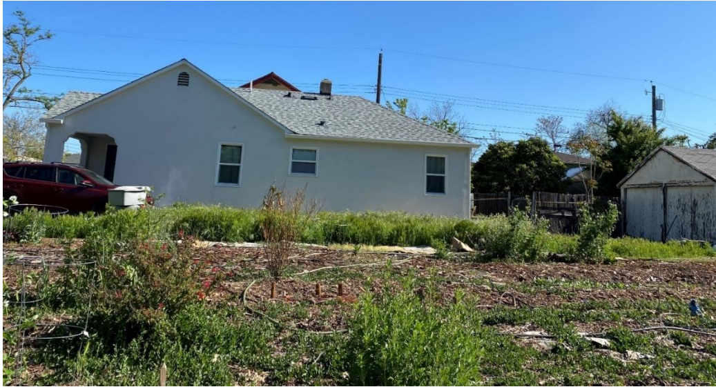
Photograph 3: Photo of south side of building. Camera facing north.
