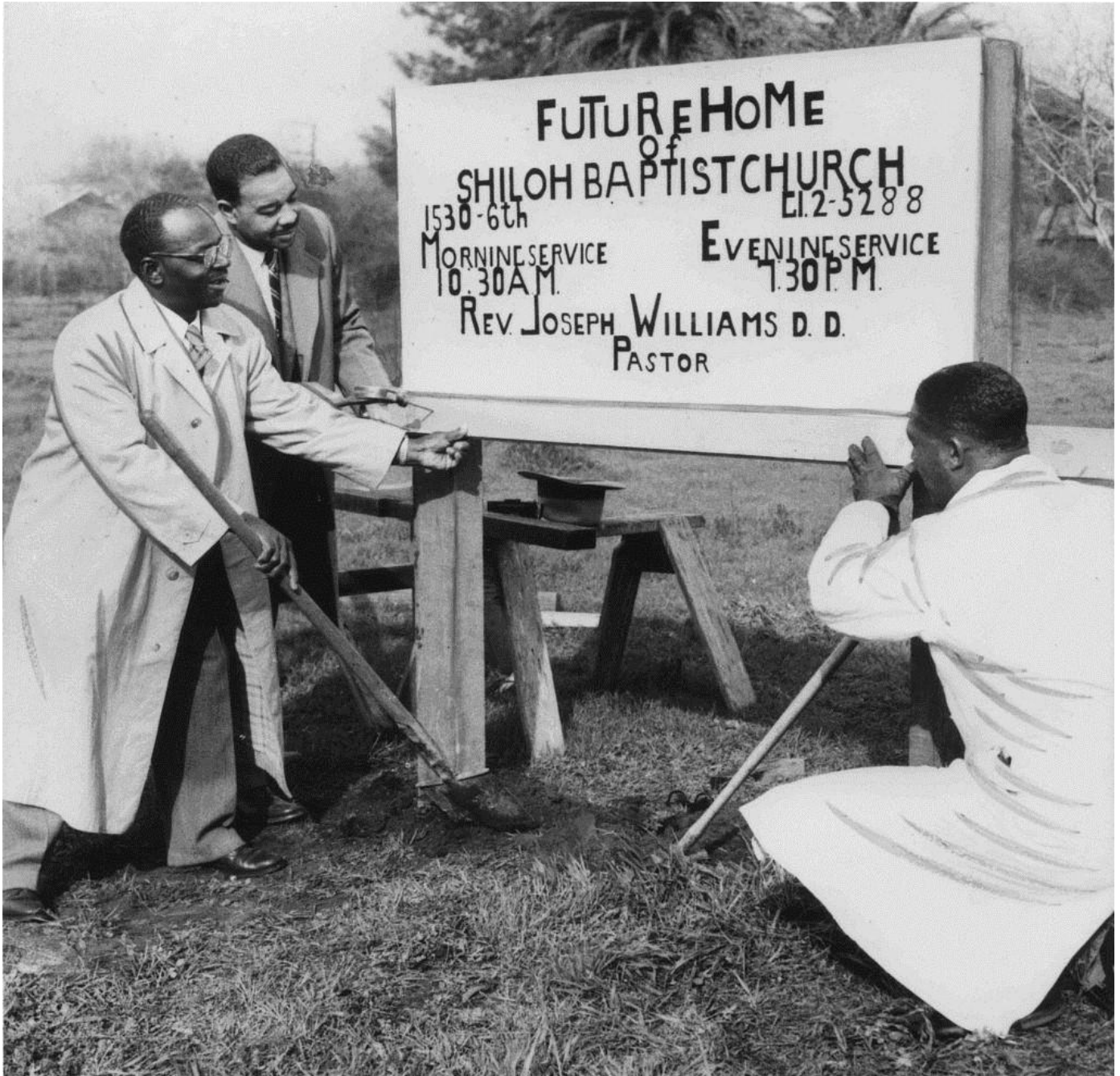
Figure 1. Groundbreaking of the new location of Shiloh Baptist Church, Rev. Joseph Williams pictured holding shovel.
