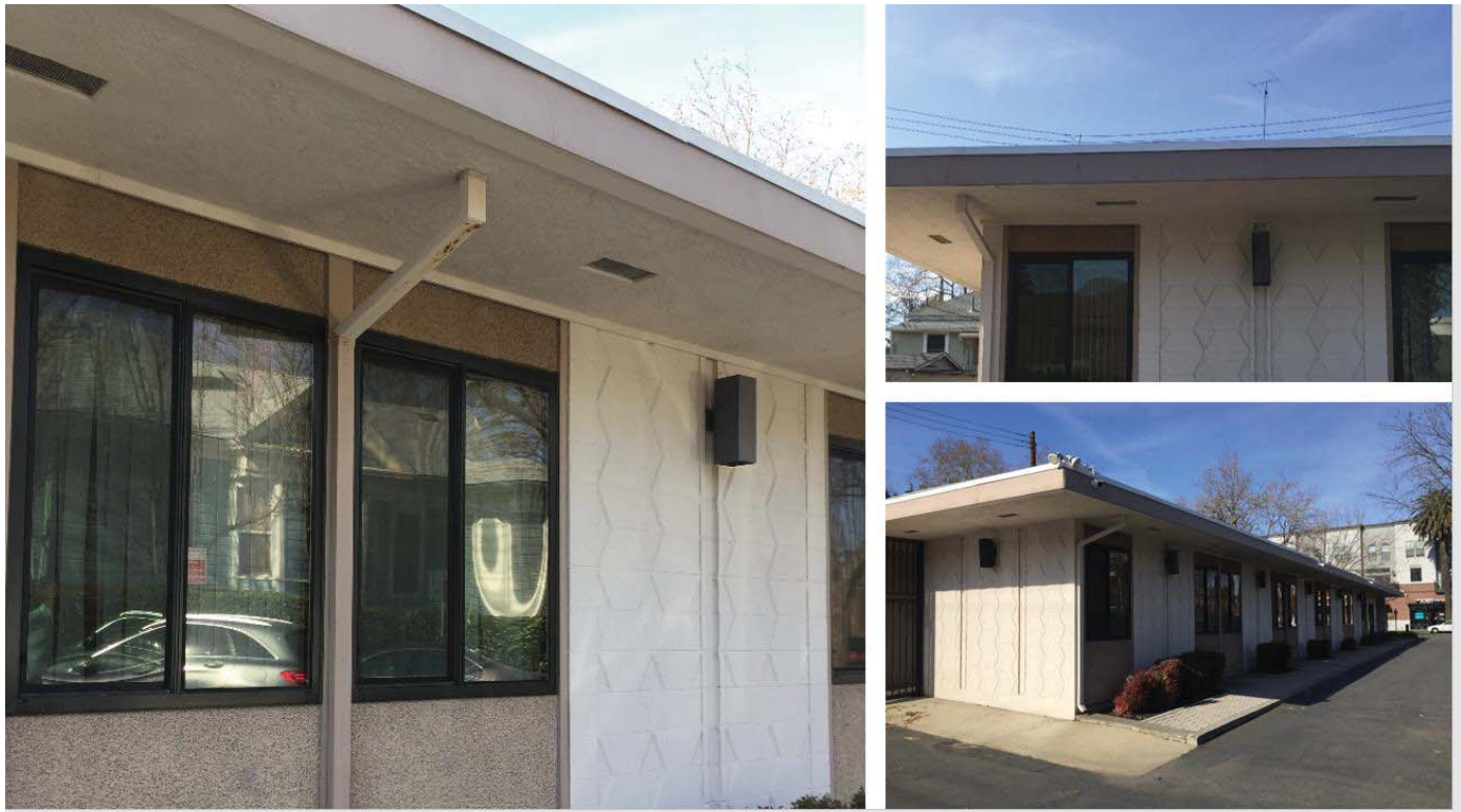
Eaves, Geometric Concrete Blocks, East Façade
