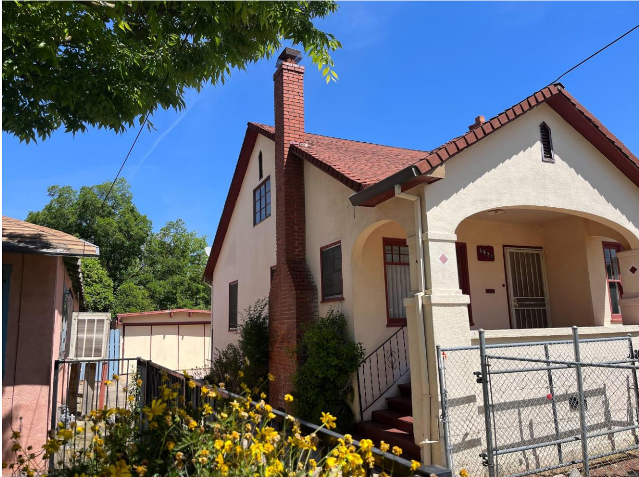
Photograph 3: West side of building, note garage and original windows.
