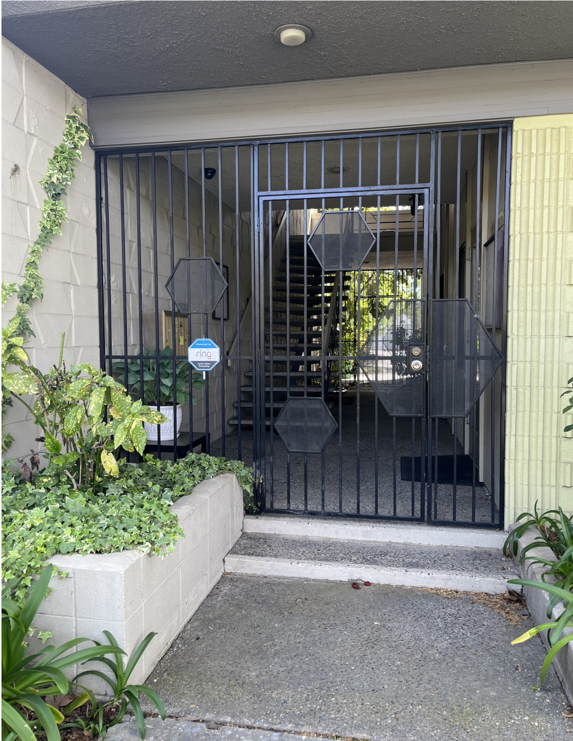
Figure 2: Photograph 3: Camera facing south depicting front entrance gate, April 23, 2023.
