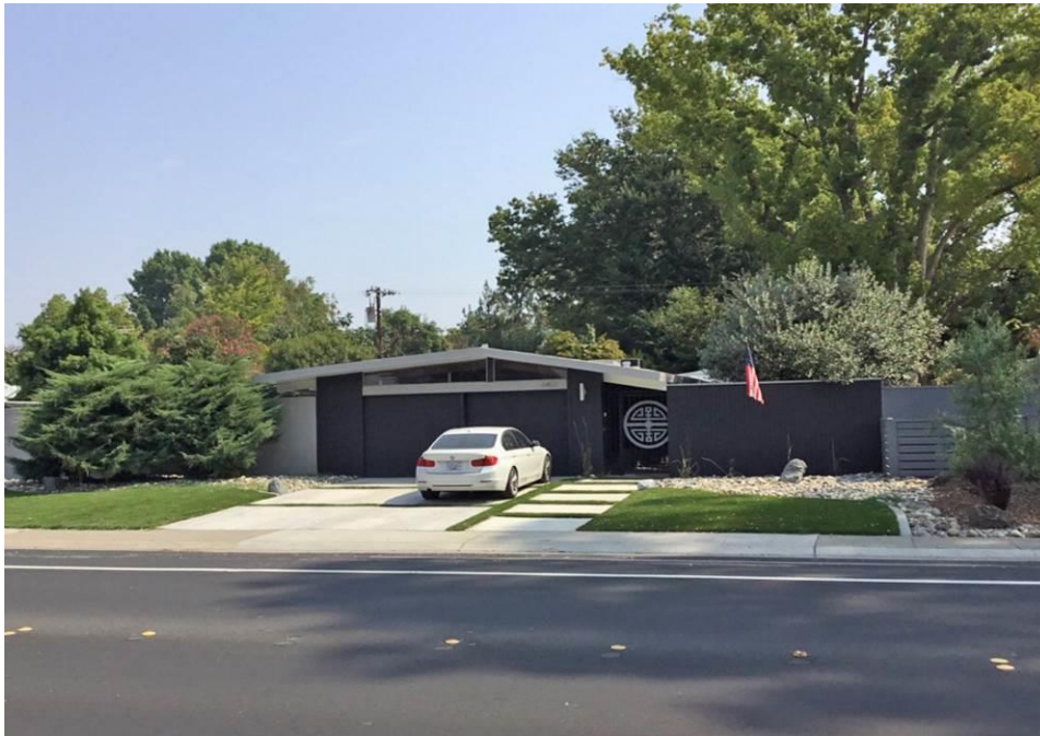
Photograph 6. 6457 South Land Park Drive, camera facing northeast September 2, 2017
