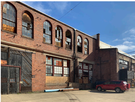
West facade of Car Shop No. 3, view southeast (ARG 2020).
