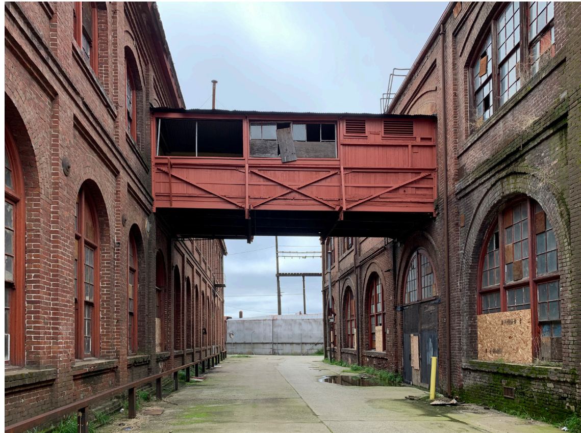
Pedestrian bridge connecting the Planing Mill (l) and Car Machine Shop (r), view west-southwest (ARG 2020).
