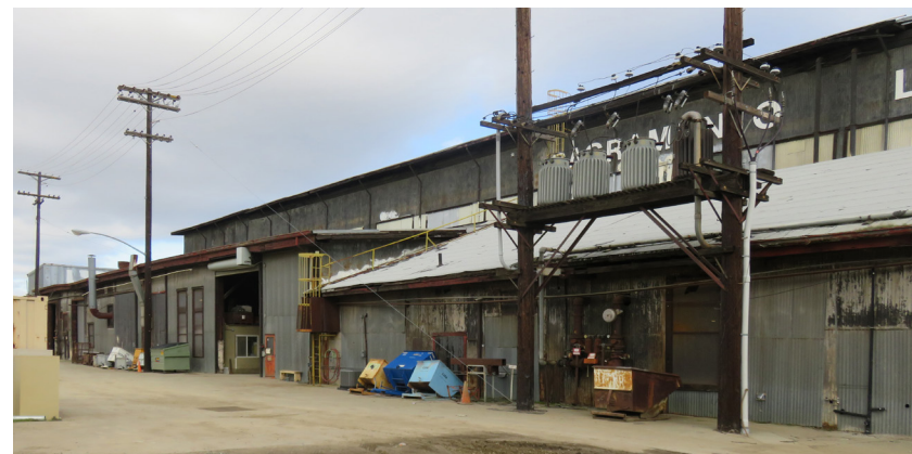
West facade of Boiler Shop, view northeast (ARG 2020).
