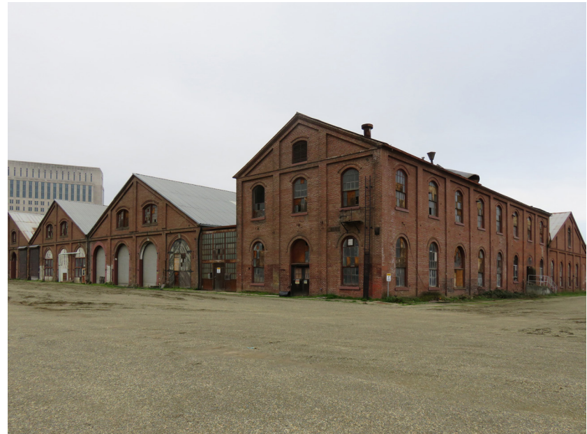
Paint Shop, view southwest (ARG 2020).
