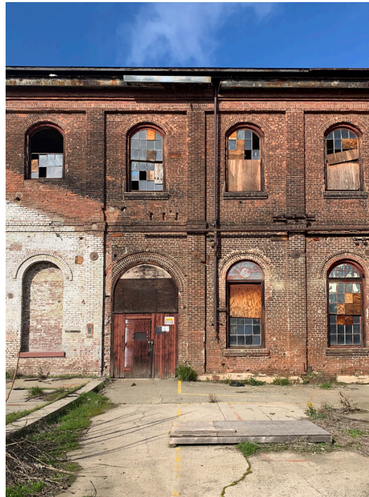
Planing Mill door, view north-northwest (ARG 2020).
