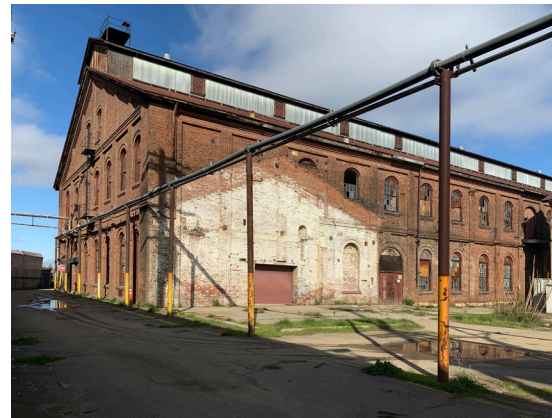
Planing Mill, showing former location of Power House, view northeast (ARG 2020).
