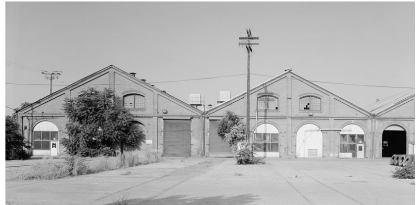
Paint Shop, view west (Historic American Engineering Record, Jet Lowe, 2001).
