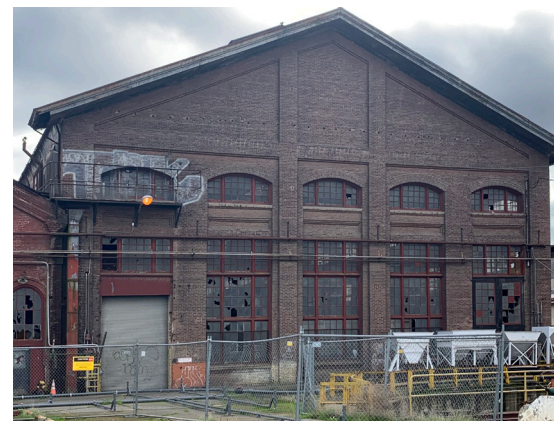
South facade of Erecting Shop, view north (ARG 2020).
