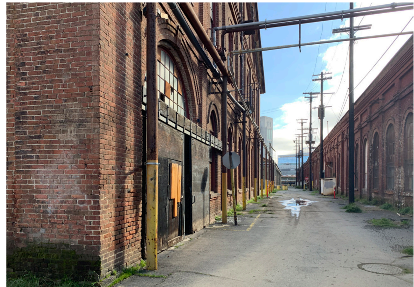
Alleyway between Planing Mill (l) and Erecting Shop (r), view south-southeast (ARG 2020).
