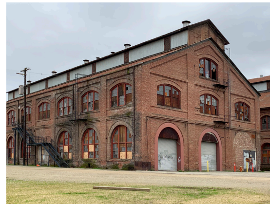
Car Machine Shop, view southeast (ARG 2020).
