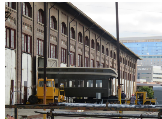
Erecting Shop and Transfer Table, view south-southeast (ARG 2020).
