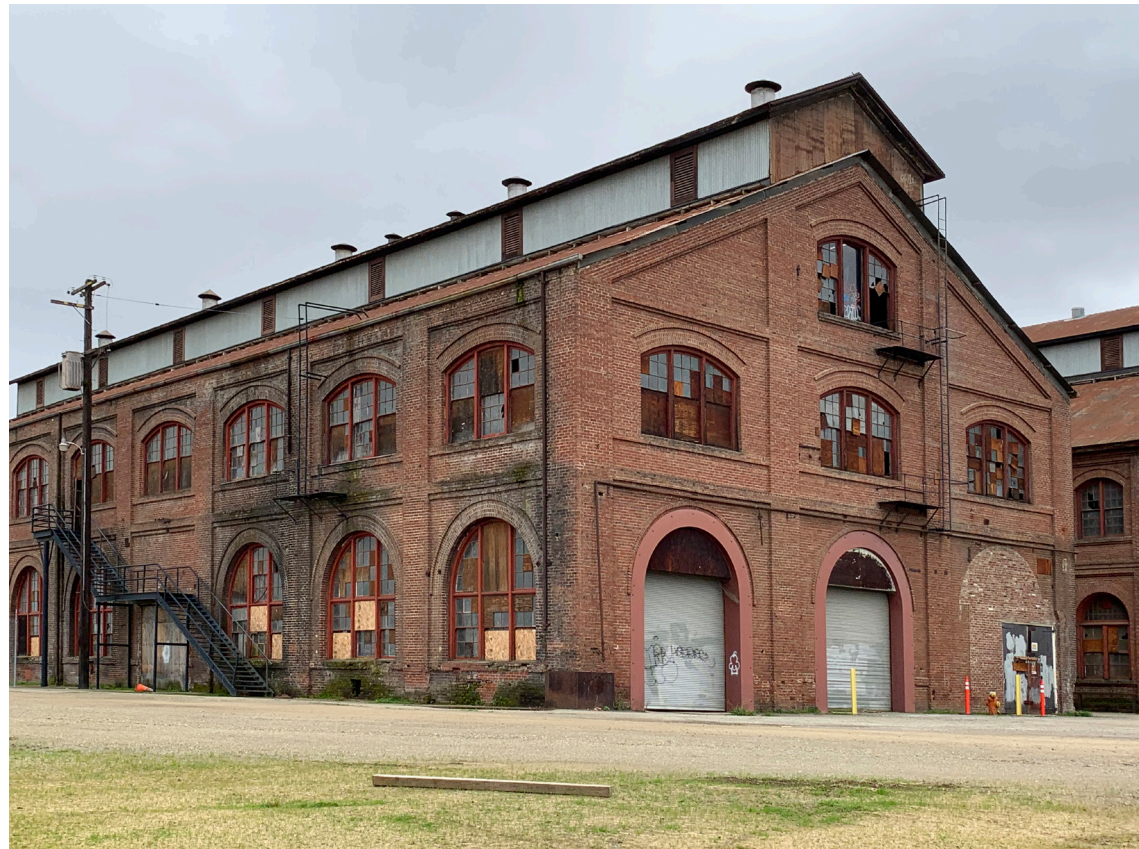
Car Machine Shop, view southeast (ARG 2020).
