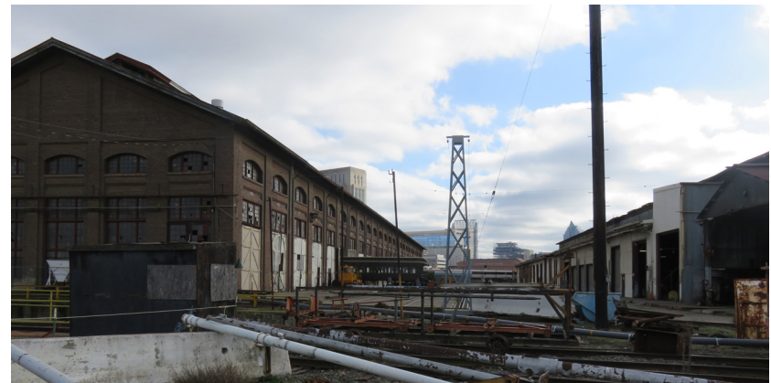
Locomotive Transfer Table, view south-southeast (ARG 2020).
