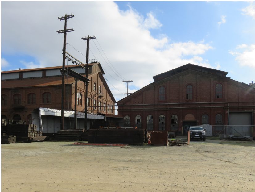
Planing Mill (l) and Erecting Shop (r), view south-southeast (ARG 2020).
