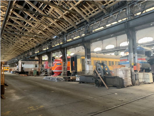
Erecting Shop interior (ARG 2020).
