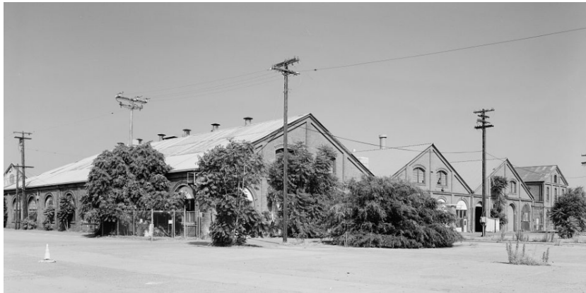
Paint Shop, view northwest (Historic American Engineering Record, Jet Lowe, 2001).
