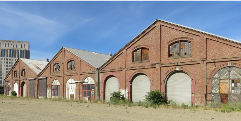
Paint Shop, view southwest (ARG 2020).
