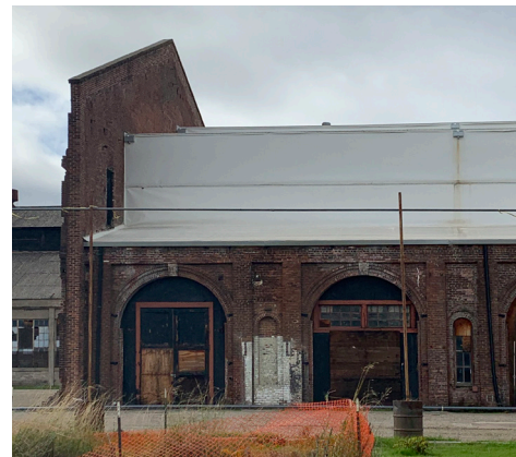
East facade of Car Shop No. 3, view west-southwest (ARG 2020).
