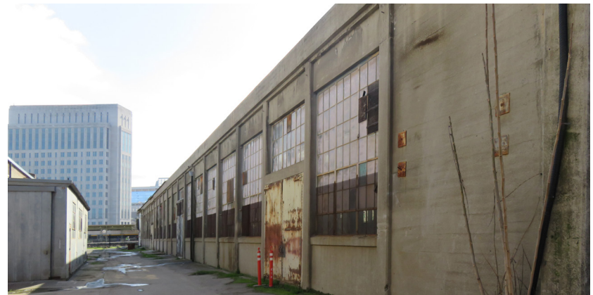
East facade of Blacksmith Shop, view southwest (ARG 2020).
