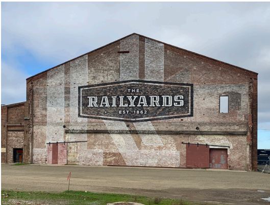
South facade of Car Shop No. 3, view north (ARG 2020).
