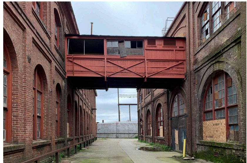
Pedestrian bridge connecting the Car Machine Shop (l) and Planing Mill (r), view east-northeast (ARG 2020).
