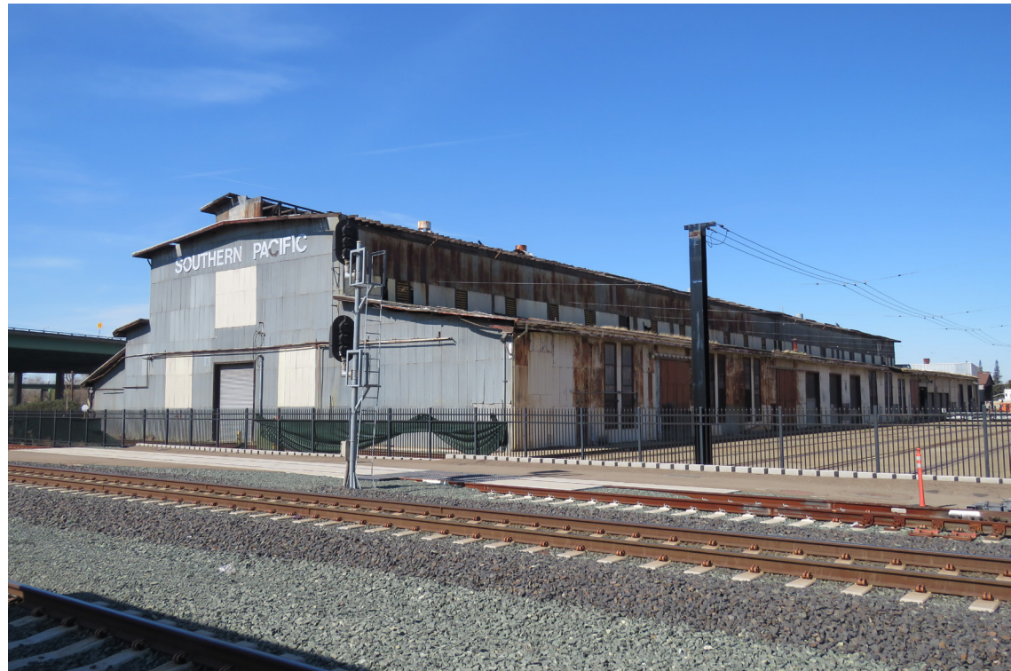
Boiler Shop, view southeast (ARG 2020).
