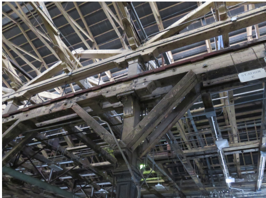
Detail of cast iron post in Erecting Shop (ARG 2020).
