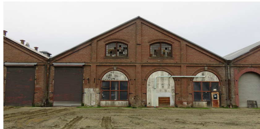
Paint Shop, view west-southwest (ARG 2020).
