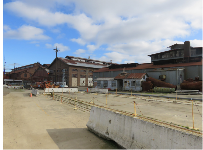
Planing Mill (l), Erecting Shop (c), Firing Line (front r) and Boiler Shop (rear r), view southeast (ARG 2020).
