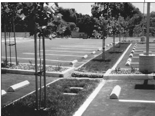
Bio-swales collect stormwater runoff and improve run-off water quality.
