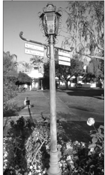
Decorative pedestrian lighting that complements nearby residential structures
