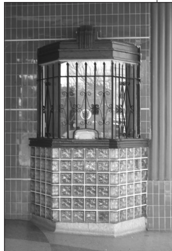
The ticket booth at the Colonial Theater, with examples of glass block and tile
