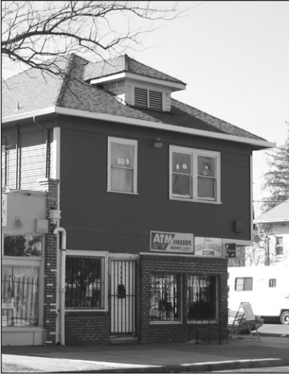
John's Philly Corner is typical of several two-story commercial structures with hip roofs and wood lap siding.
