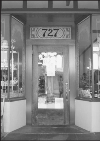
A traditional recessed entry with stained glass transom.
