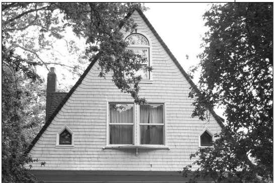
Steeply pitched, front-facing gable roof
