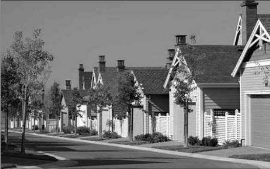
Reduced alley aprons decrease pavement runoff.
