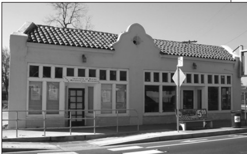
California Mission Revival is a common architectural style in the Stockton Commercial Character Area.
