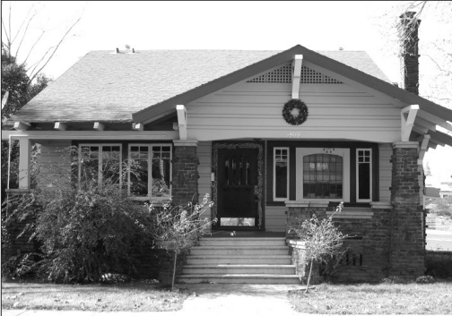
This bungalow has the front crossing gable and triangular knee braces under the eaves typical of the style.
