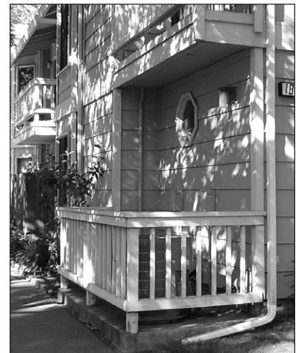
Appropriate screening of HVAC unit behind fence
