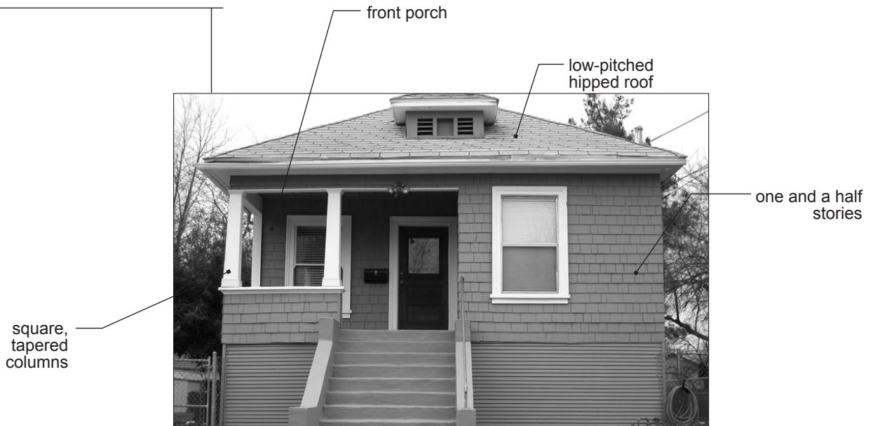
Sacramento Highwater Bungalow with raised main story
