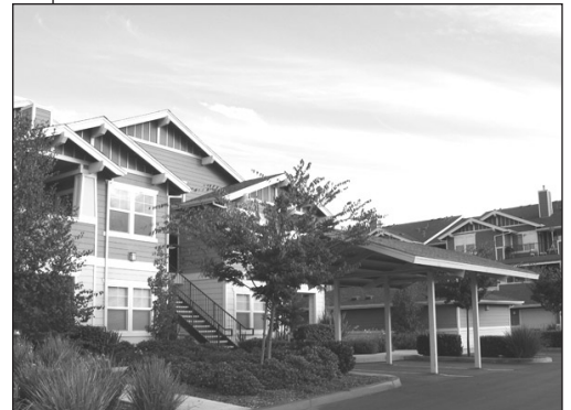
Parking is in small, dispersed lots in the interior of this multi-family development. The materials on the carport also match those on the main buildings.
