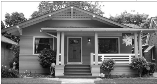
This entry feature adds dynamic interest to an older home in the Residential Character Area.
