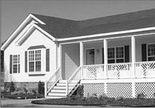
This manufactured home has been constructed with brick over the foundation and a front porch to give the appearance of permanency.
