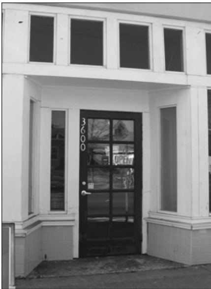
This recessed entry shows the oversized wooden window framing found on some older buildings on Stockton Boulevard. (For a view of the entire building, see page 70.)
