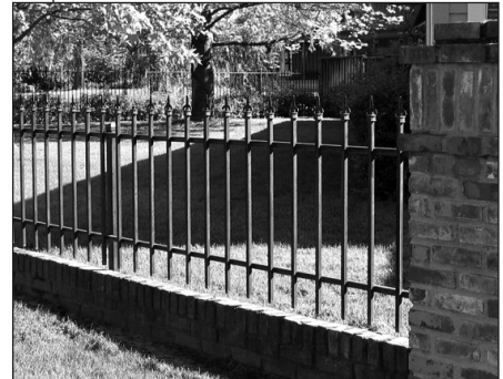
Brick and metal mixed materials
