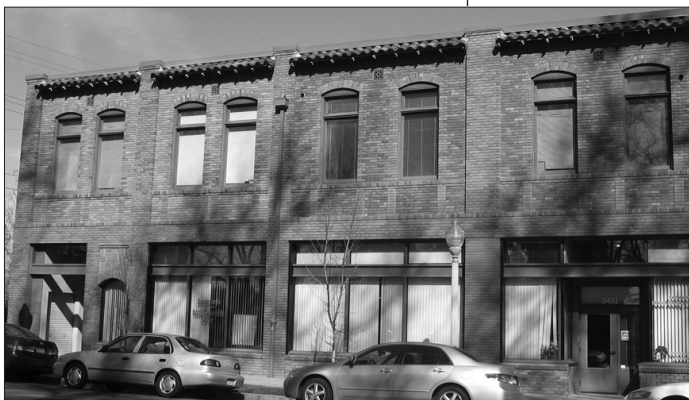
Upper floor windows in the Broadway Commercial Character Area should be vertically proportioned.
