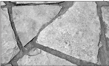
Flagstone mortared on concrete
