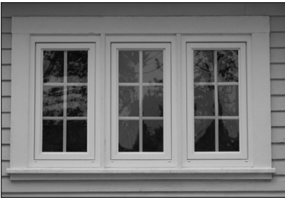
Casement window with wooden frame and sills
