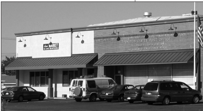
Steel overhangs help to articulate commercial entries, offer shade and add architectural interest to the building.
