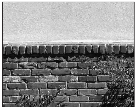
Brick wainscoting on smooth stucco
