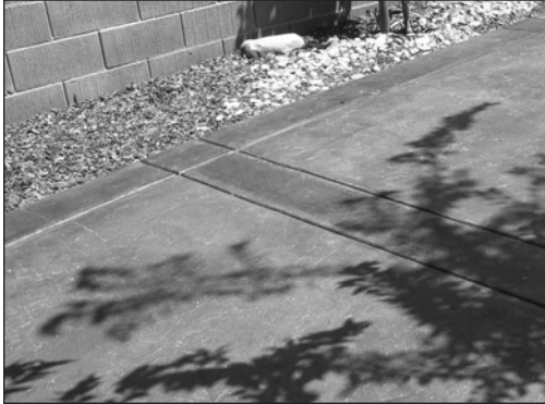
Concrete paving can be enhanced with detailing and the use of integral color.
