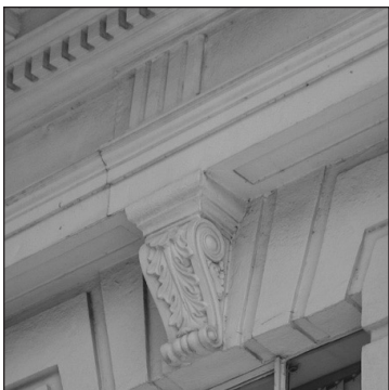
Terra cotta detailing
