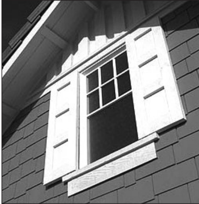
Window detailing, such as shutters, adds interest.
