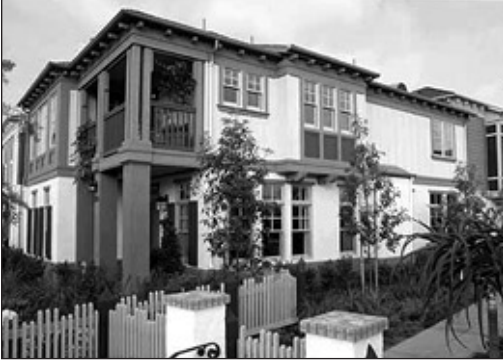
A multi-family structure with defined entries, gates, and paths.
