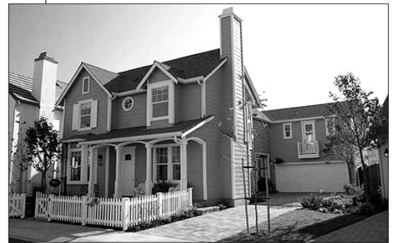
Attached garage recessed from the front facade of the home
