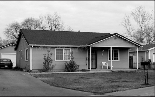
Relatively larger front yard setbacks are typical of some homes south of South Avenue.
