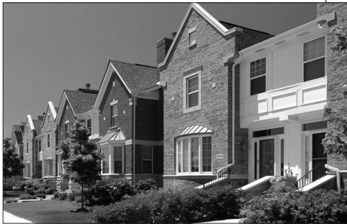
Bay or bow windows can help to articulate a residential facade as exemplified in these two-story duplex units.
