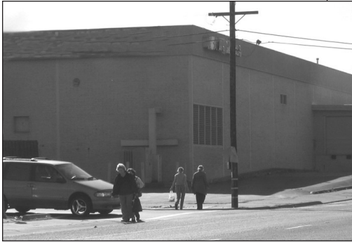
Avoid expansive blank walls along streets.
