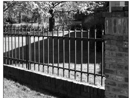
Metal fence with brick column
