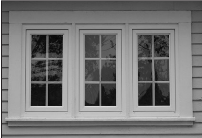
Casement window with wooden frame and sill
