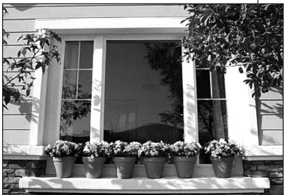
Attractive window detailing
