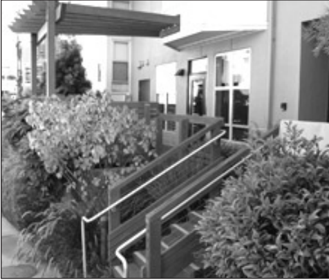
Landscaped entry area, steps, and a small porch have been constructed for each unit in this multi-family structure.
