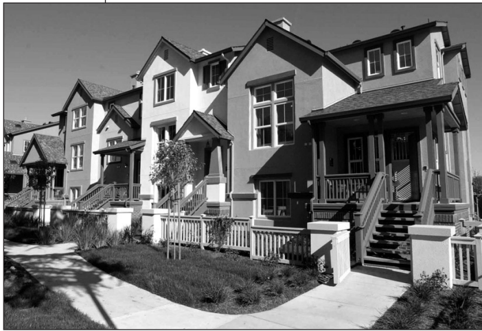
These townhomes have facade details and colors that distinguish them as individual units.
