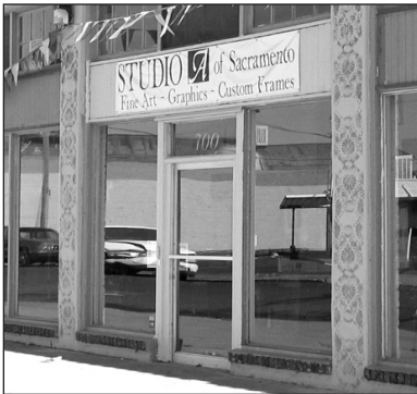
Even simple entries can be embellished with architectural detailing to improve their appearance. This building has decorative painted trim.
