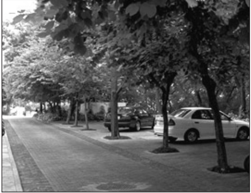
The interlocking pavers in this shaded parking lot help to keep stormwater runoff on-site.
