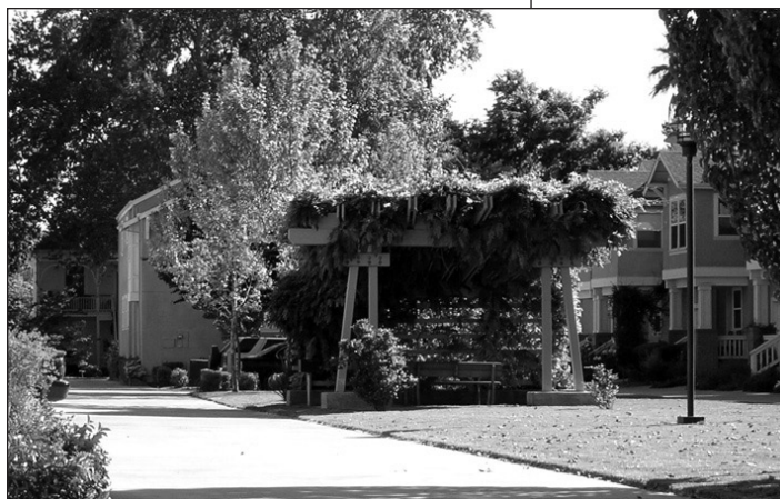
This multi-family complex has an inviting interior common space with picnic area.
