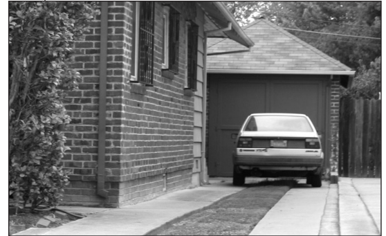
Detached garage at the rear of a home
