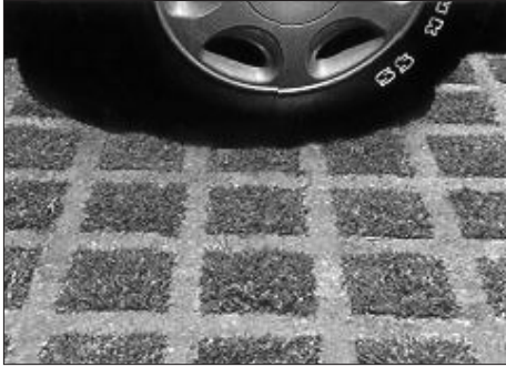
Alternative surfaces such as grass pavers keep stormwater runoff on-site and reduce heat production.
