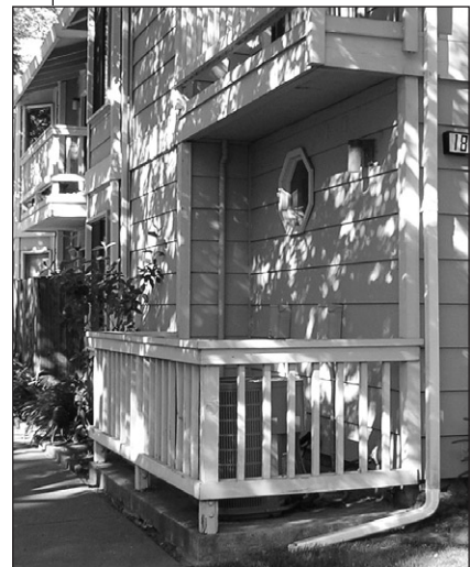
Appropriate screening of HVAC unit behind fence
