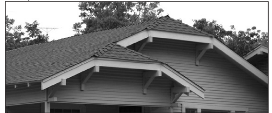
Gable roof with clipped end
