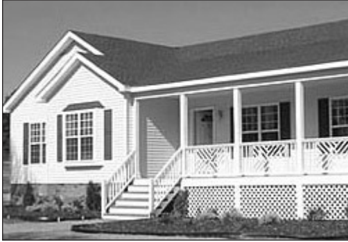
This manufactured home has been constructed with brick over the foundation and a front porch to give the appearance of permanency.
