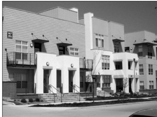
This contemporary multi-family development has been designed with setbacks similar to adjacent commercial development.
