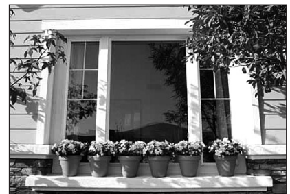
Attractive window detailing Photo Courtesy of DesignLens
