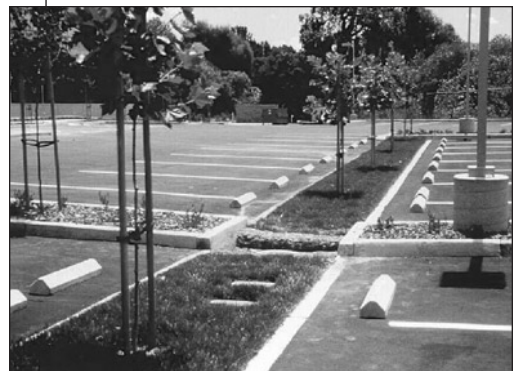
Bio-swales collect stormwater runoff and improve run-off water quality.
