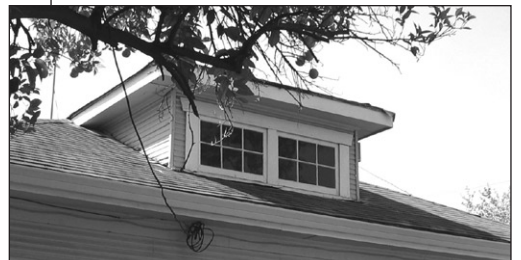
Dormer windows and other decorative roof elements help to break up the mass of a two-story home.
