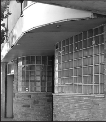
Glass block can be found in some older buildings in North Sacramento, and may be used in small amounts in infill and renovations.
