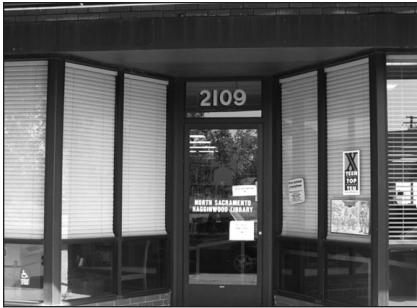
This recessed entry on the public library is typical of many older buildings on Del Paso Boulevard.
