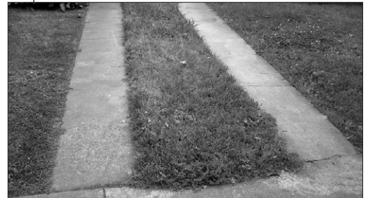
Alternative driveway materials, such as turf strips, can minimize the amount of paving in driveways.
