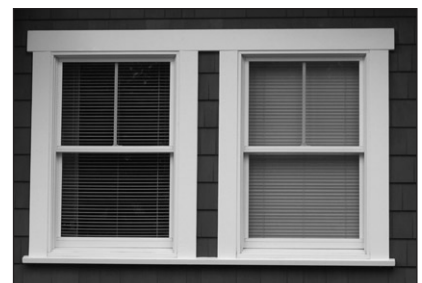
Single-hung windows with wooden frame
