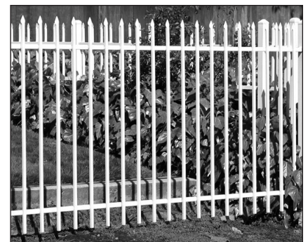
Metal fence with ornamental top condition
