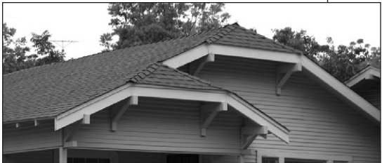
Gable roof with clipped end
