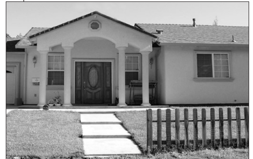
This front yard setback on an infill home in North Sacramento is designed to meet current City standards.
