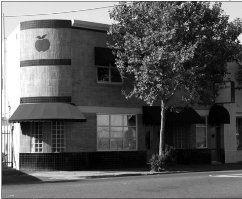
Renovated Streamline Moderne building
