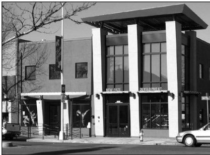
New Faze on Del Paso Boulevard has a dramatic corner feature with a street level entry opening onto the pedestrian way.
