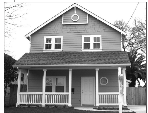
Entry clearly visible and single-story porch proportional to the home
