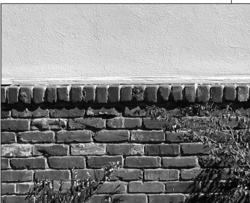
Brick wainscoting on smooth stucco
