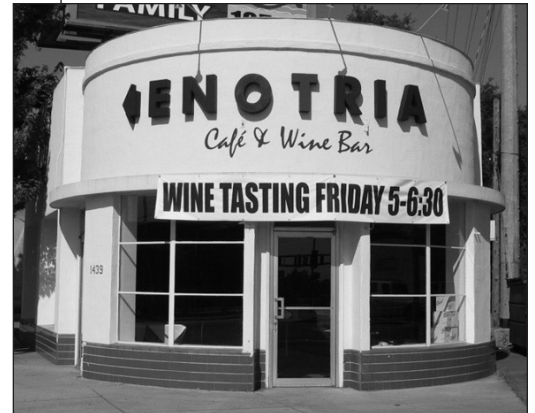
Renovated corner entry on Del Paso Boulevard
