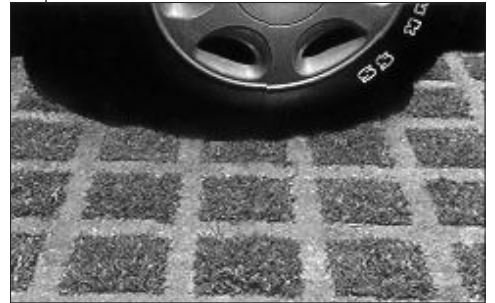
Alternative surfaces such as grass pavers keep stormwater runoff on-site and reduce heat production.
