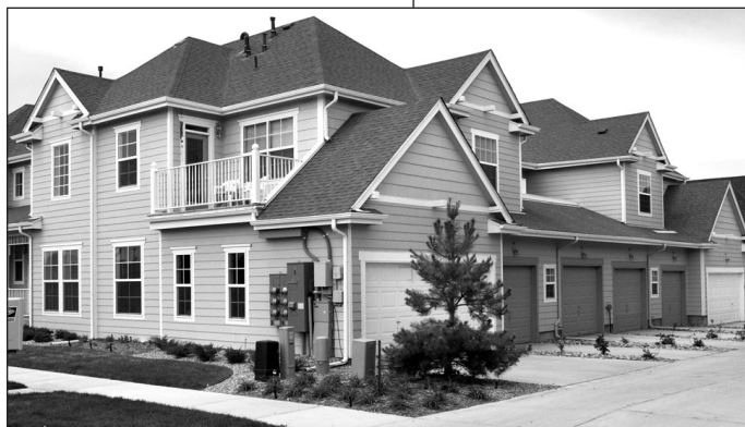
The garages are located at the rear of this multi-family structure.
