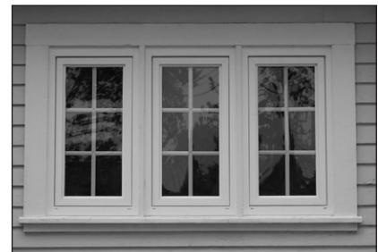
Casement window with wooden frame and sill
