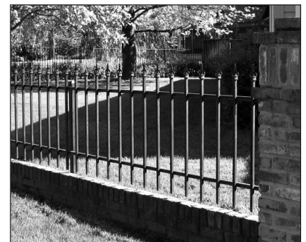
Metal fence with brick column
