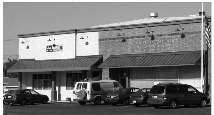
Steel overhangs help to articulate commercial entries, offer shade, and add architectural interest to the building.
