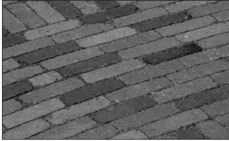
Brick set on sand and gravel base
