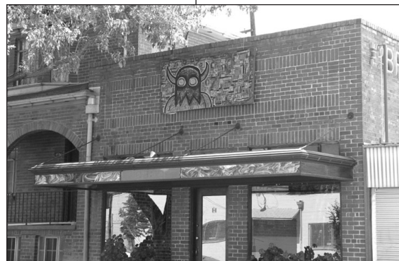
Typical flat commercial roof
