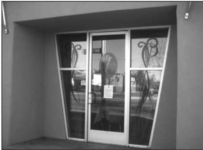
The Supper Club has a more contemporary recessed entry and door.
