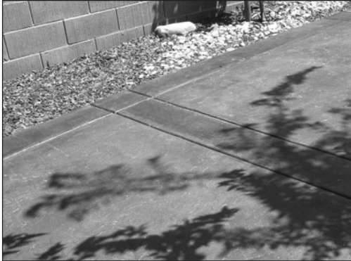
Concrete paving can be enhanced with detailing and the use of integral color.
