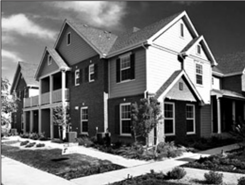
These multi-family homes have been designed with setbacks and architectural features similar to those found in single-family homes.
