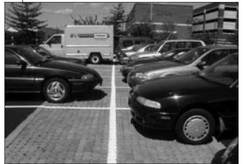
Modular pavers are another attractive alternative that helps to keep stormwater runoff on-site.
