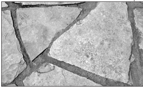
Flagstone mortared on concrete
