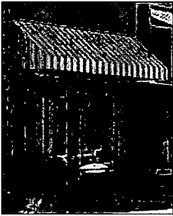
Awnings on south facing windows can reduce heat gain.
