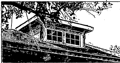
Dormer windows and other decorative roof elements help to break up the mass of a two-story home.
