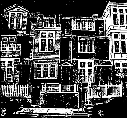
This three-story row house development sets the third floor back and has a facade that is complementary to nearby single-family homes.
