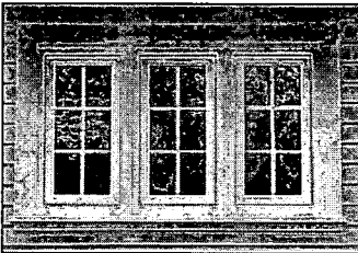
Casement window with wooden frame and sill
