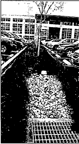
Bio-swales collect stormwater runoff and improve run-off water quality.
