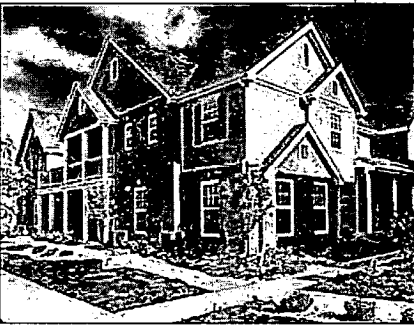
These multi-family homes have been designed with setbacks and architectural features similar to those found in single-family homes.
