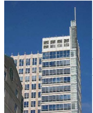
Bulk reductions and integrated mechanical penthouses contribute to the distinctive tops of these Sacramento towers.
