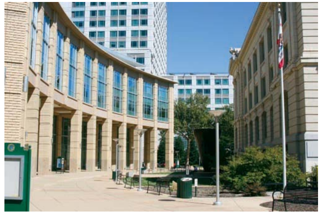
New development that is designed in a manner that is respectful of an adjacent historic structure.
