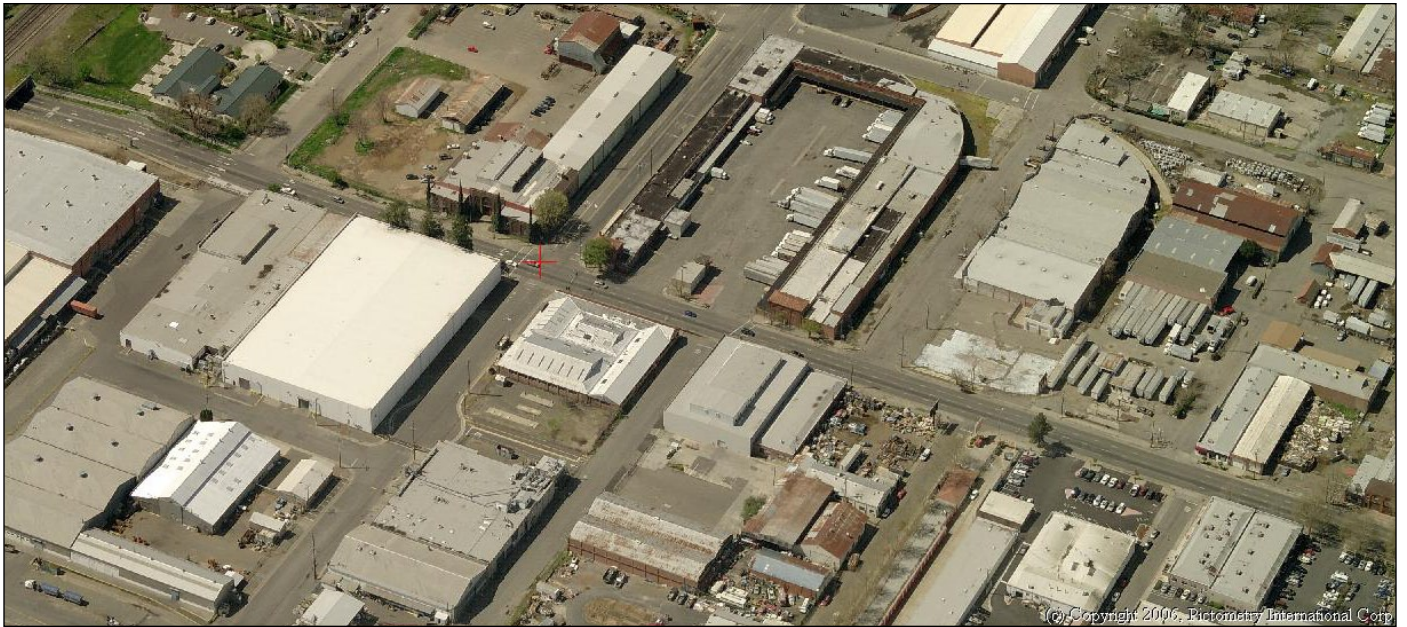
Figure 2.98. This aerial view of North 16th Street and the surrounding area illustrates the unique building form and the potential for infill development and adaptive reuse of many existing buildings.
