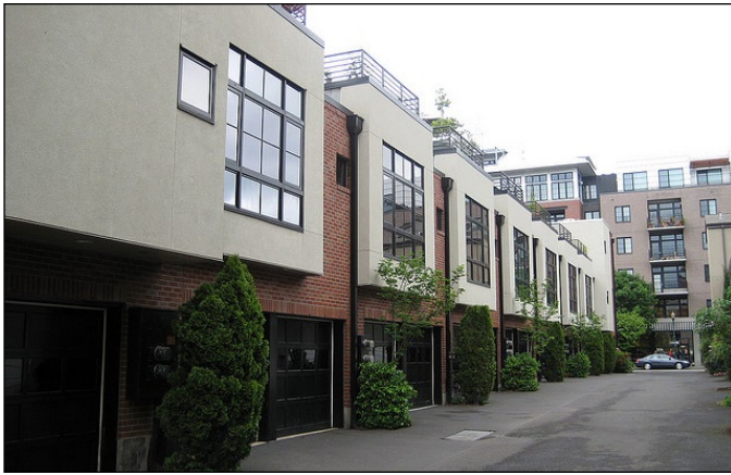
Figure 2.84. Residential uses which back onto alleys can mediate the utilitarian purpose and enhance security with landscaping and strong visual connection to the alley.
