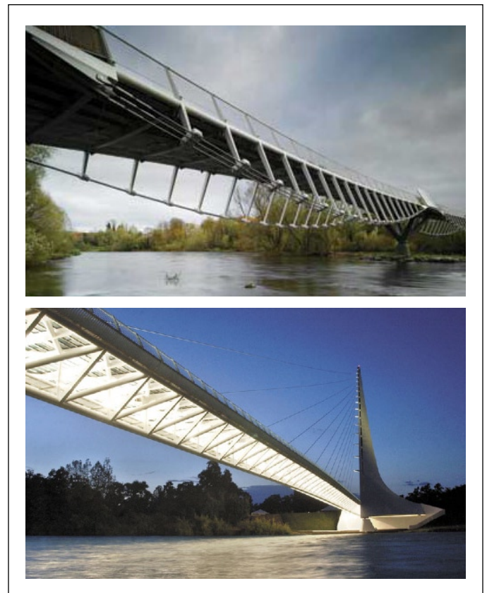
Figure 2.44. Artful bridges can give identity to a place or region while respecting the natural environment. The Living Bridge on the River Shannon, Ireland (above) and the Sundial Bridge in Redding, California illustrate how structure and light can be used to move beyond simple utilitarian infrastructure where the natural beauty of the surrounding should be complimented.
