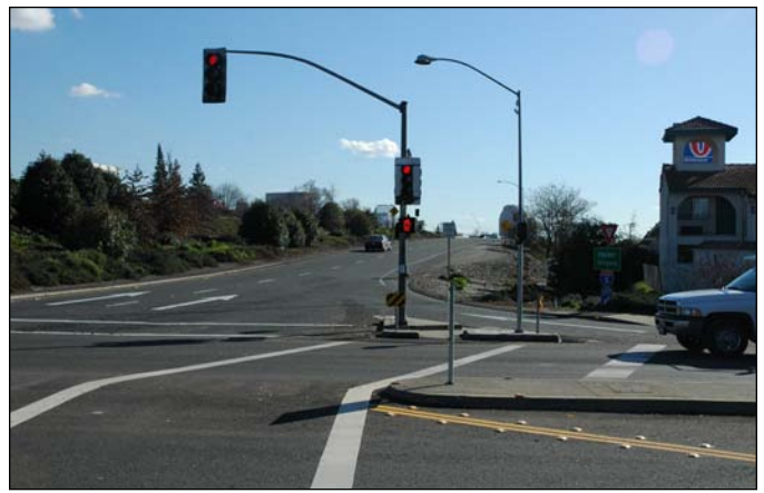
Figure 2.50. Freeway access at Interstate 5 and the lack of pedestrian facilities design results in the isolation of the Jibboom Street Area from the remainder of the district.
