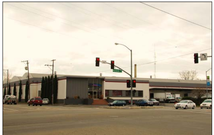
Figure 2.79. The Sacramento Theatrical Company building at Richards Boulevard and 10th Street is an impressive long span curved-truss building.
