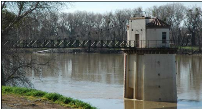
Figure 2.57. An example of civic infrastructure in the grand tradition, the City of Sacramento Water Intake Facility provides exceptional public viewing of the Sacramento River along its perimeter balcony.
