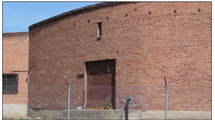
Figure 2.100. Several buildings in the area were built to the curvature of rail-road spur lines that give the area a distinctive architectural character.
