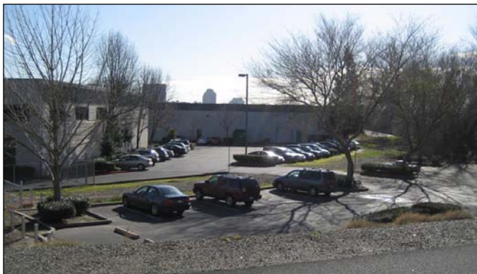
Figure 2.63. View from the levee shows the typical site planning in the area with parking and storage areas adjacent to levees and buildings facing inward.
