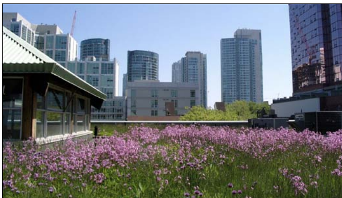
Figure 2.8. Roof gardens in dense urban areas provide visual relief while decreasing roof heat loads, filter run-off and abate storm water surcharges.
