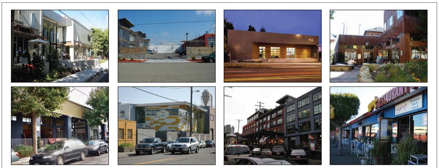
Figure 2.95 Reuse of warehouse buildings in the Dos Rios Street Area should explore creative solutions and celebrate eclectic design integration.
