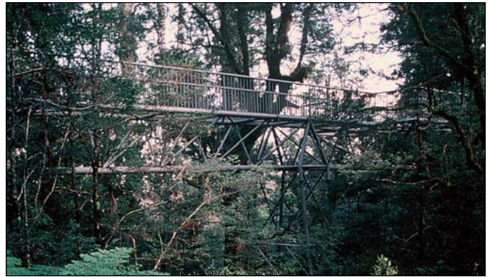
Figure 2.43. Lightweight spaceframe structure provides access into the rain-forest jungle in southern Australia. The structure is supported from a single column support.
