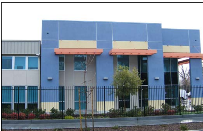
Figure 2.78. Low-rise office buildings recently added to the area.
