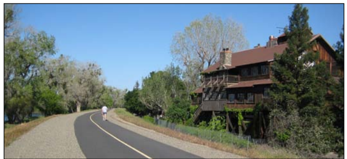
Figure 2.39. This former restaurant is the only structure along the American river to take advantage of the views to the American River Parkway.
