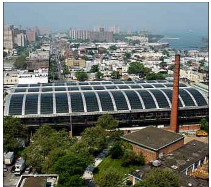
Figure 2.10. Solar photovoltaic panels cover the roof of a transit station in New York City is similar in profile to some warehouses in the River District.
