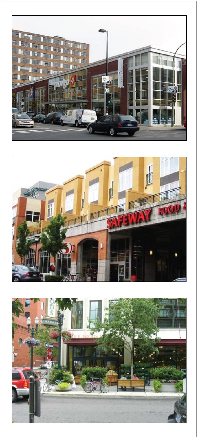
Figure 2.71. Three urban grocery store examples which illustrating mixed use integration and urban standalone markets which engage the streetscape. Top to Bottom: Provigo, Quebec, Canada; Safeway, Seattle, WA; Whole Foods, San Francisco, CA
