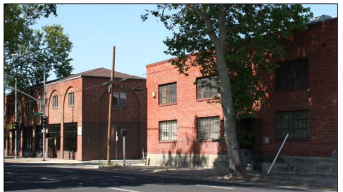
Figure 2.102. The brick masonry buildings along North 16th Street exist in a corridor that can be enhanced with new streetscape and street parking.
