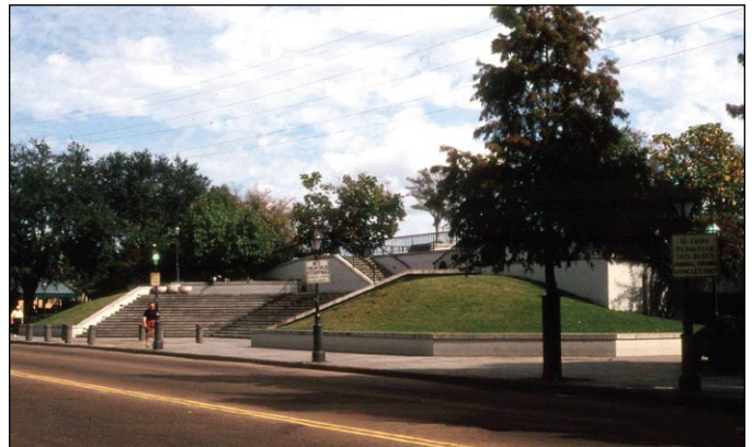
Figure 2.12. New Orleans Washington Artillery Park steps leading to levee embankment of the Mississippi River.
