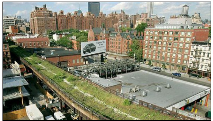
Figure 2.23. New York's new elevated parkway along abandoned subway line.
