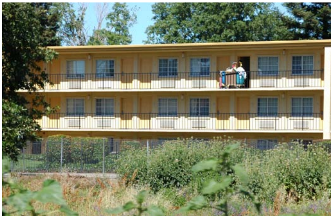
Figure 2.49. 1970's era motels along the Sacramento River do not take full advantage of the river views or the opportunity to create a riverfront hospitality destination. (Luis Alvarado Photo)
