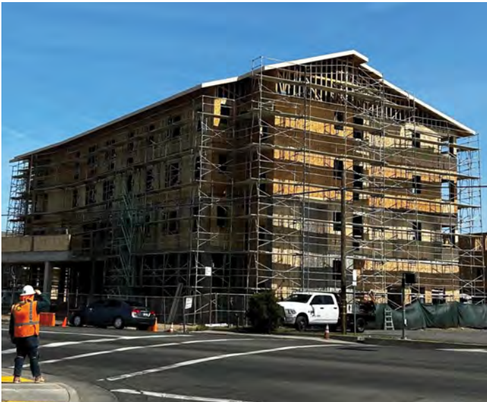
Housing construction in the Specific Plan Area.
