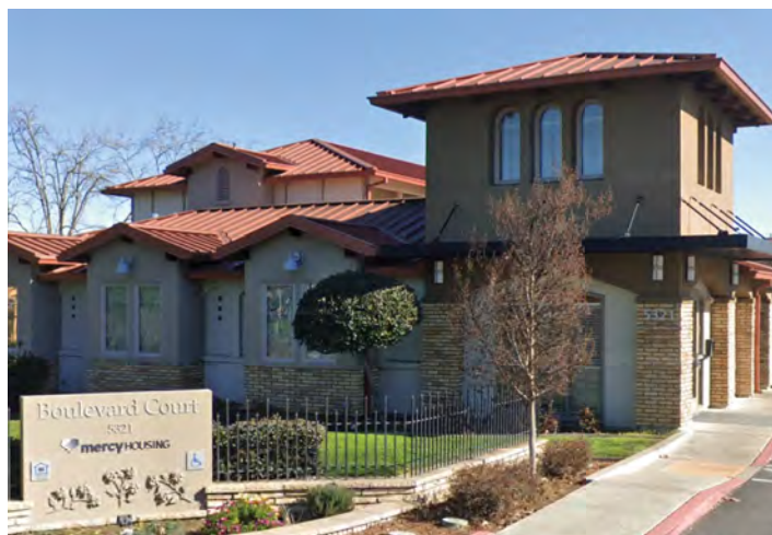
Residential uses, such as this affordable housing complex, account for only 8 percent of the land on the corridor.
