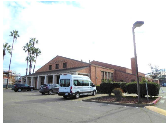
Figure 19. Governor's Hall at the intersection of Stockton Boulevard and Broadway.
