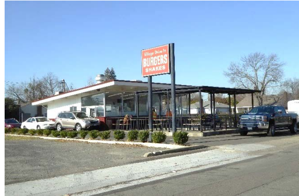
Figure 31. The Village Drive-in at 3810 60 th Street.
