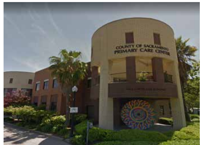
Office uses account for nearly 15 percent of the land on the corridor.
