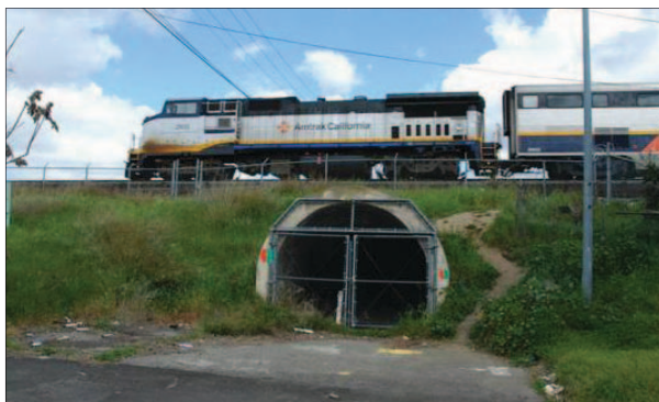
FIGURE 5.8 North 14th Street Tunnel, Closed in 1994.
