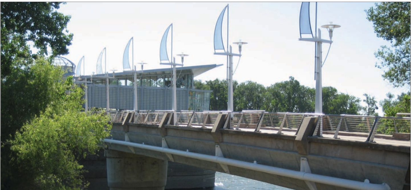
FIGURE 2.0 Sacramento River Water Intake Facility.
