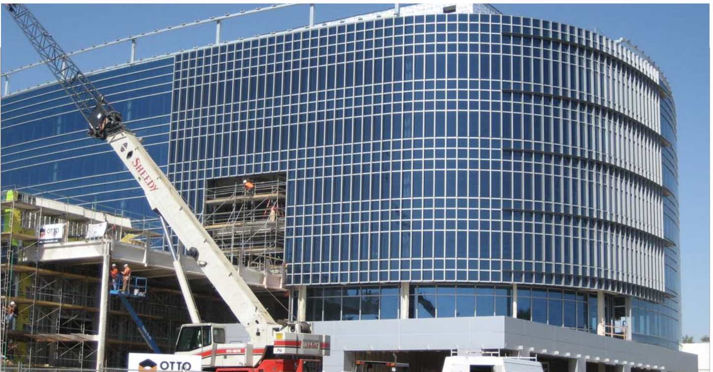
FIGURE 3.0 Lottery Headquarters under Construction, 2010.
