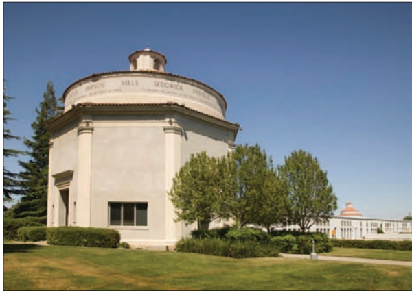
FIGURE 8.2 Sacramento Historic Water Treatment Building.
