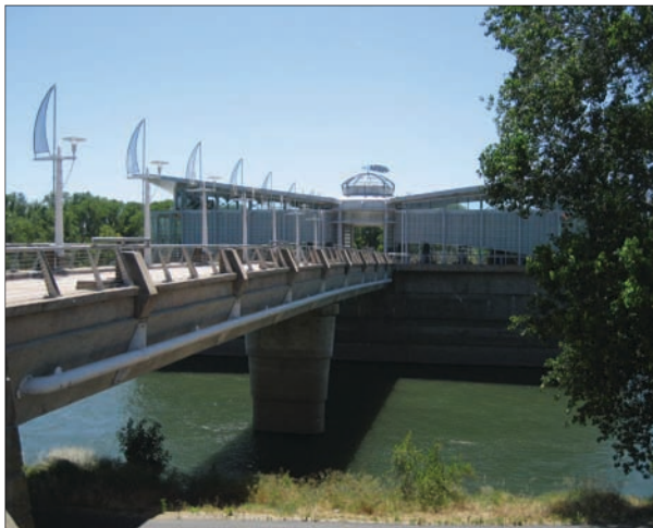
FIGURE 8.3 Sacramento River Water Intake Facility.
