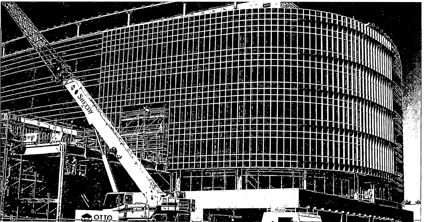
FIGURE 3.0 Lottery Headquarters under Construction, 2010.
