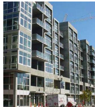
Figure 4-121 A wide street frontage is articulated with bay windows, projecting balconies, and recessed zones. The major massing articulations begin above the 2nd floor.
