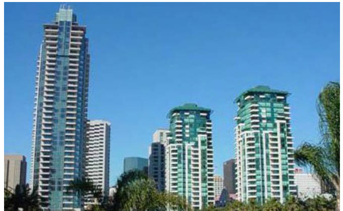
Figure 4-84. High-rise residential buildings- shown here in downtown San Diego- typically have minimal ability to accommodate stepback recommendations, due to the requirements for residential units to "stack" in a repetitive fashion. Massing articulations are often found in balcony and terrace configurations.
