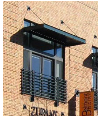
Figure 4-155. French balcony covering windows & operable doors
