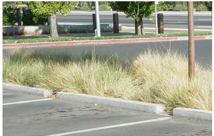
Figure 4-248. Sustainable storm-water management: parking area drains to bioswale rain garden.
