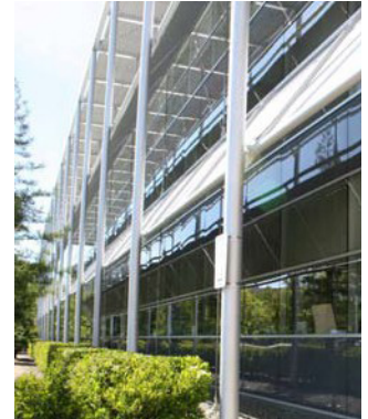
Figure 4-148. Applied sun shading elements on a building at Stanford University, Palo Alto, CA.
