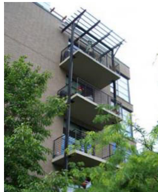
Figure 4-154. Stacked balconies on an apartment building
