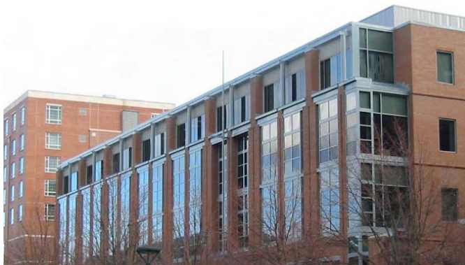
Figure 4-137. This university building in Cambridge, MA, has a repeating double window bay module which sets a rhythm across the façade, which is then interrupted by special conditions at the corner and above the entry.
