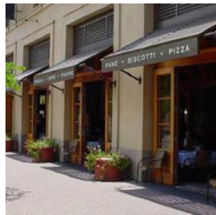
Figure 4-149. Awnings projecting over the right-of-way at ground-level retail.
