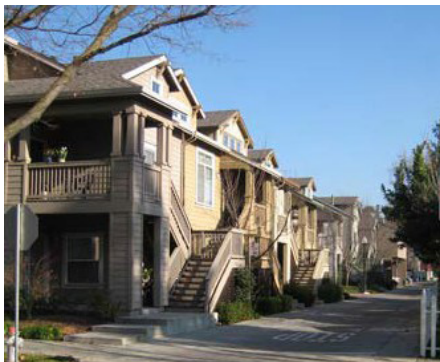
Figure 4-185. Redevelopment along Kondos Alley, Sacramento, with raised porches, stairs, and vehicular and pedestrian access.
