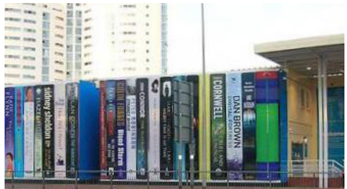
Figure 4-184: The temporary construction screening for the new City of Cardiff (Wales) Library depicts giant book spines.
