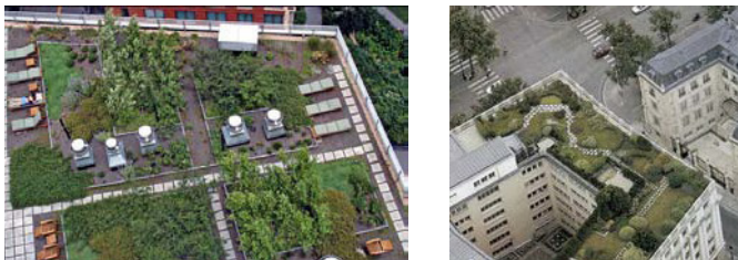
Figures 4-201 and 4-202. Green roofs can also be used as open space, can facilitate stormwater management, and reduce energy consumption by keeping a building cooler.
