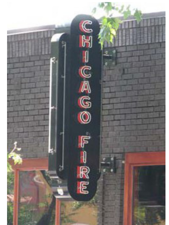
Figure 4-180. New blade sign with classic exposed neon further defines building details.
