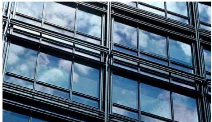
Figure 4-138. This office building at 560 Mission Street in San Francisco has a sophisticated system of projecting mullions and framing members, establishing an intricate dialogue between structure, skin and appendage.
