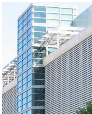
Figures 4-239 and 4-240. Parking structure at City Hall in San Jose, CA, uses horizontal metal louvers (left) and perforated metal panels (right) to control the glare produced by night lighting.
