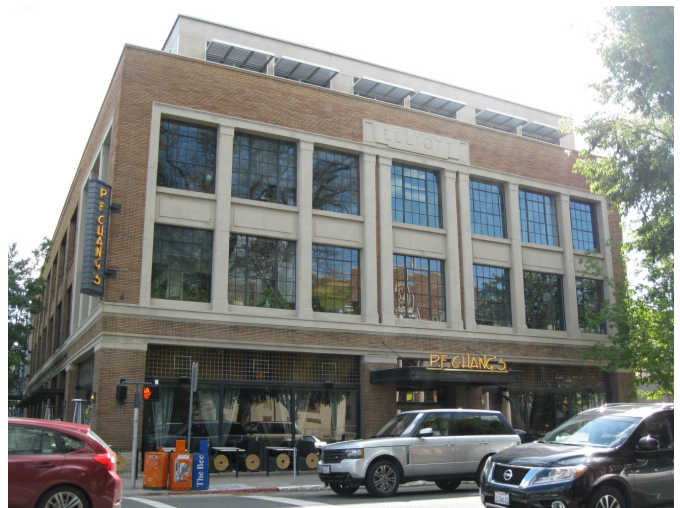
Figure 4-257. W.I. Elliott and Company Building
