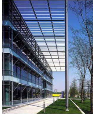
Figure 4-195. Giant canopy applied to a commercial office building, Chiswick Park, London,
