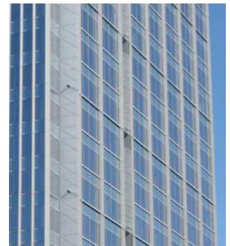
Figure 4-122. The facade of 621 capitol Mall has horizontal articulation every three floors, and a notch running vertically from top to bottom.
