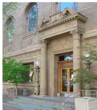
Figure 4-145. Entrance to the city library, appropriately designed and decorated.
