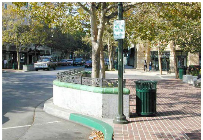
Figure 3-28. Curb extensions expand the pedestrian realm, slow traffic and reduce pedestrian crossing distance
