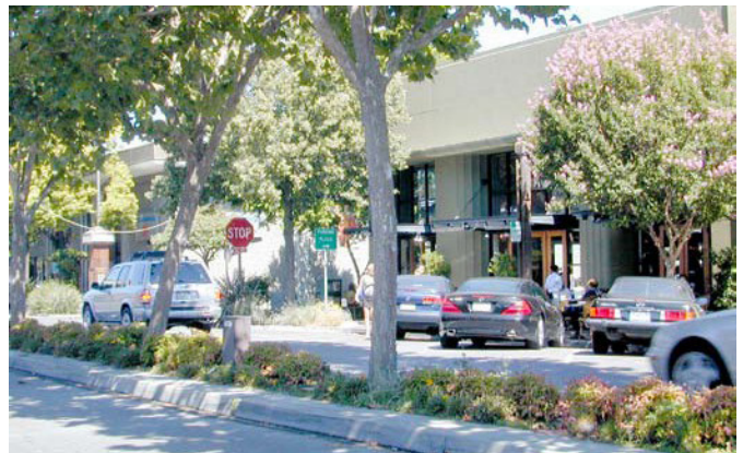
Figure 3.76. Permeable pavement and rain gardens provide stormwater management benefits (Portland, OR).
