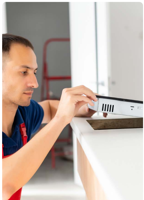
Induction Stove Installation
