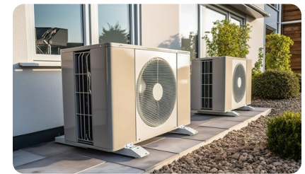
Heat Pump HVAC : Cost analysis assumes variable stage air source heat pump.
