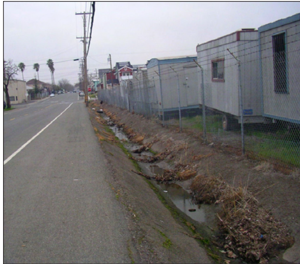
Poor storm water conditions along Dixie Avenue
