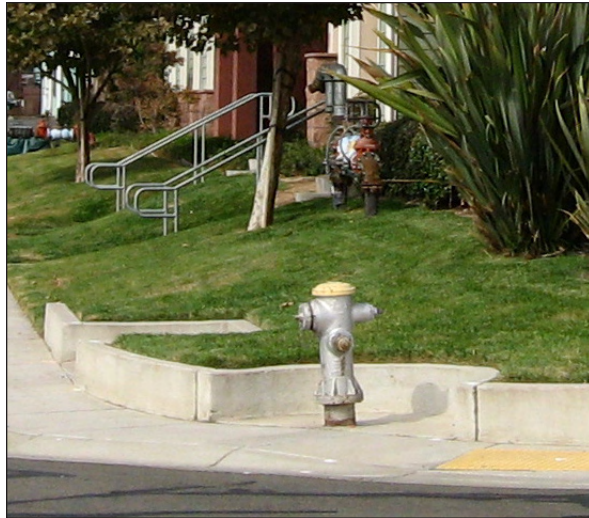
Inadequate fire protection
