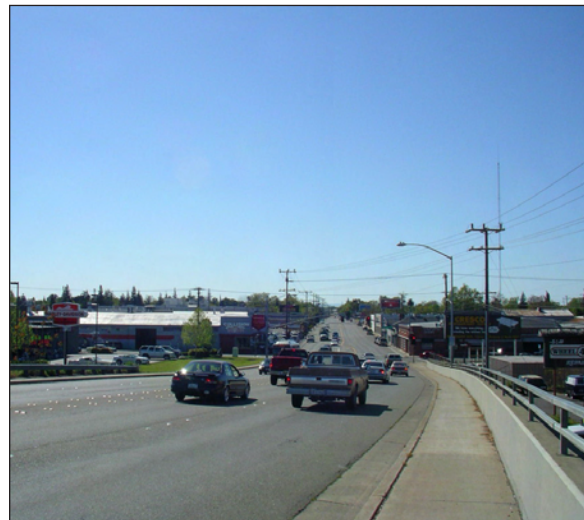
Narrow and unprotected sidewalks along Arden Way overpass
