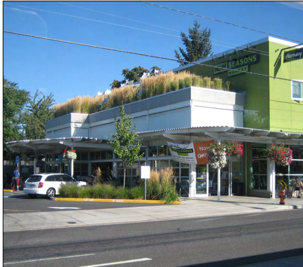
2Axi-7, 2Axi-8 Green roof on a supermarket in Portland, OR
