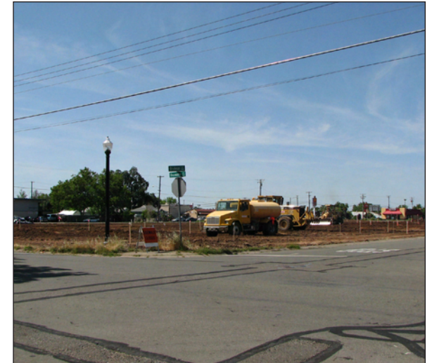
New development along Dixie Avenue
