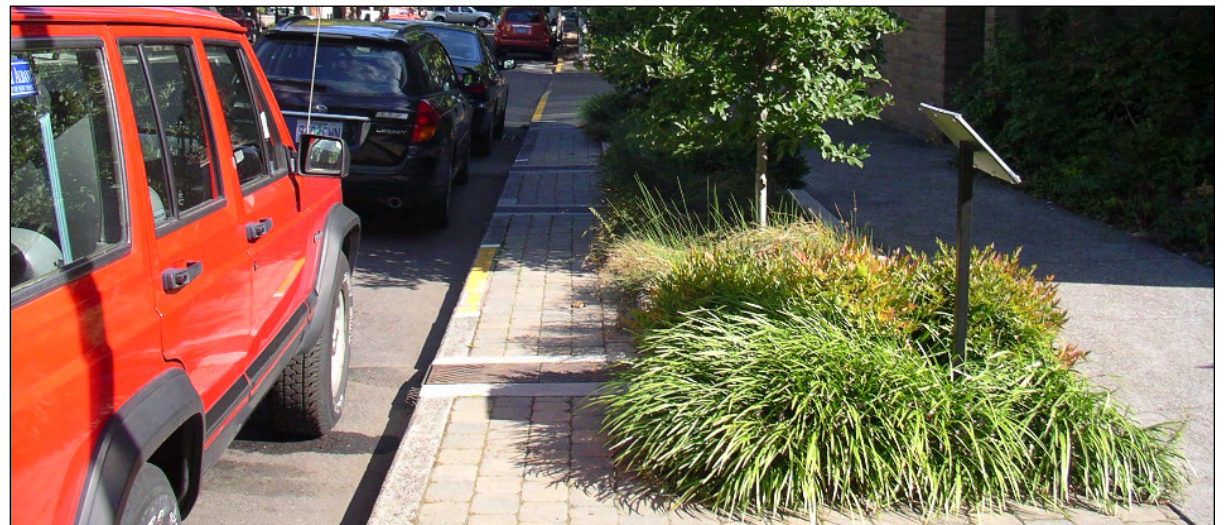
Separation between parking space and stormwater planter
