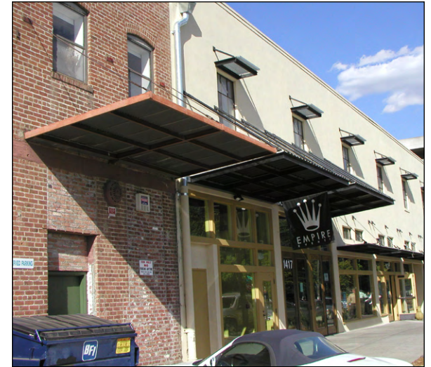
Deep overhangs on live-work units
