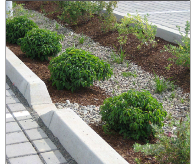
2Axi-15 Vegetated swale for treatment and infiltration
