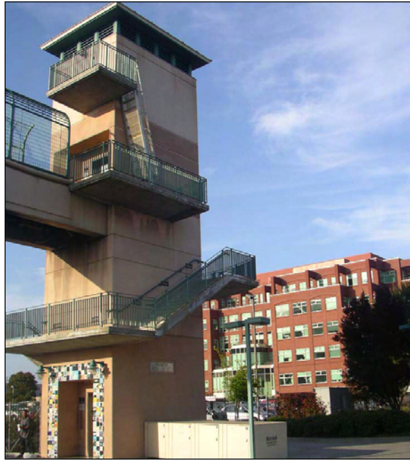
Pedestrian bridge in Emeryville, CA
