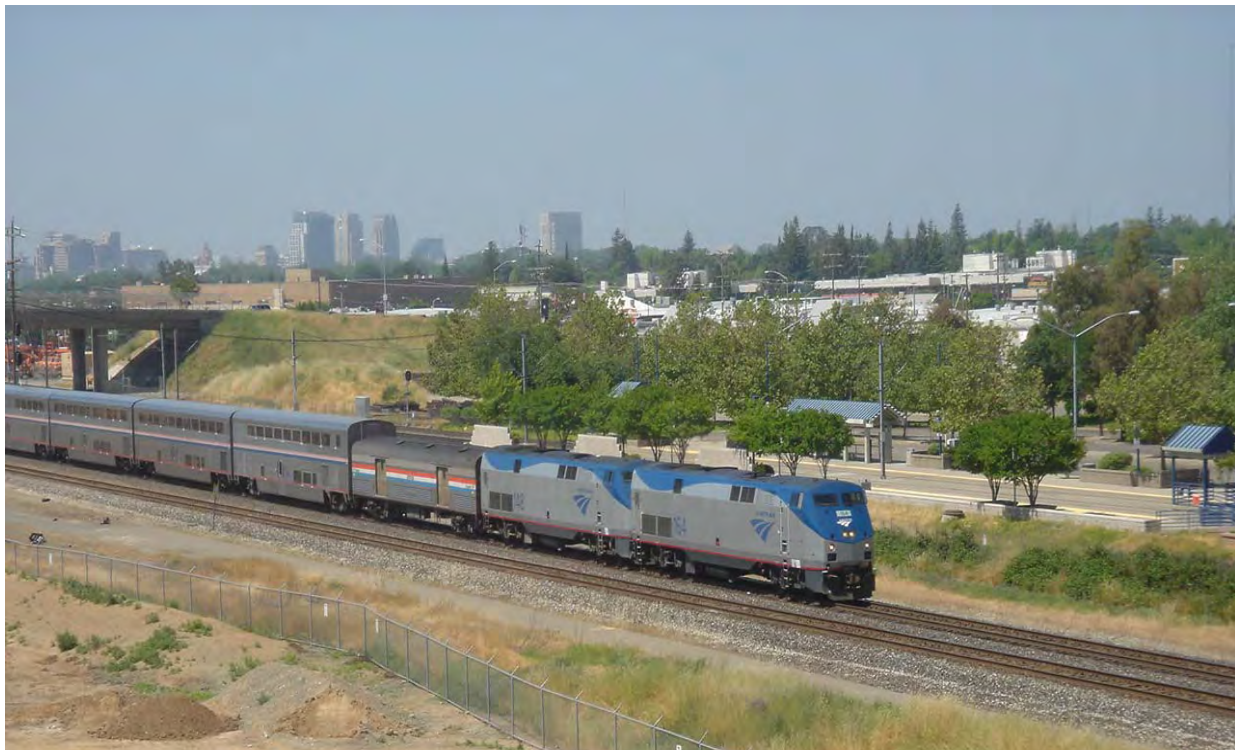
View of the station area and Downtown from the top level of the USAA parking structure
