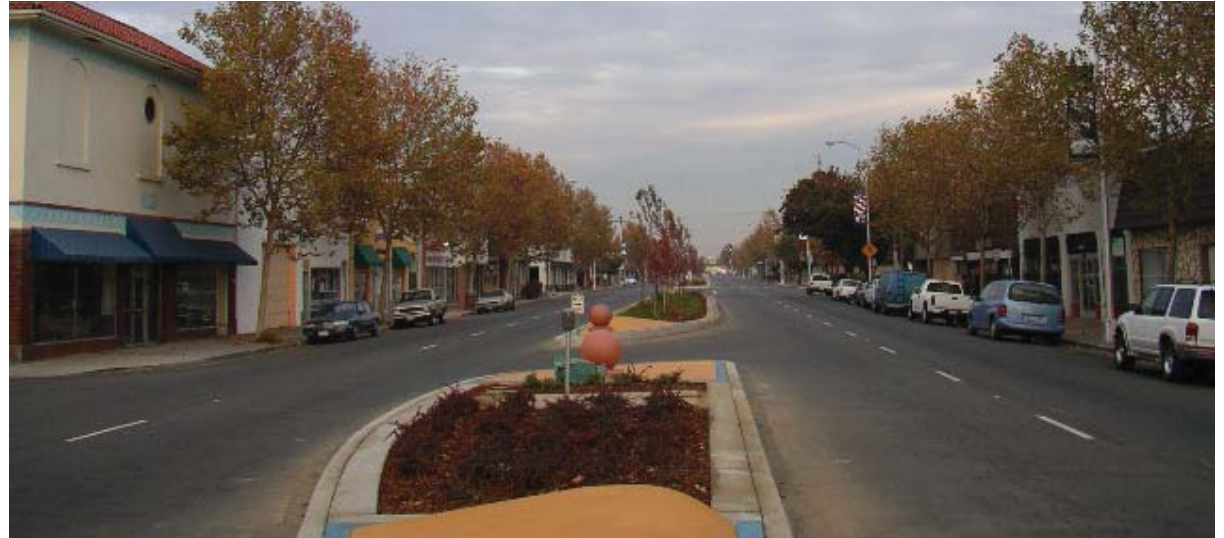
New streetscape improvements to Del Paso Boulevard
