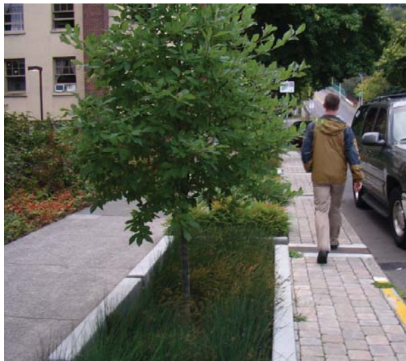
Example of integrated storm water planter area
