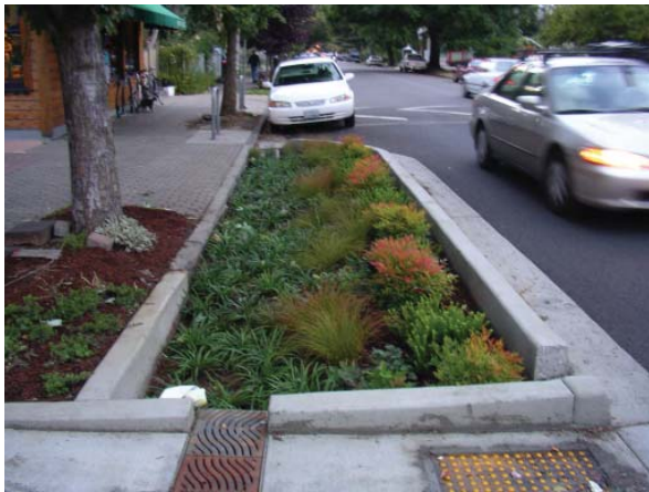
Integrated stormwater solutions along streetscape
