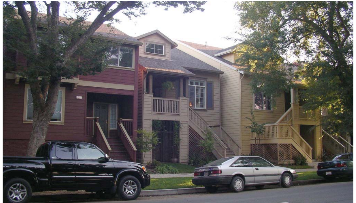
Pedestrian friendly environments along higher intensity residential development next to transit station
