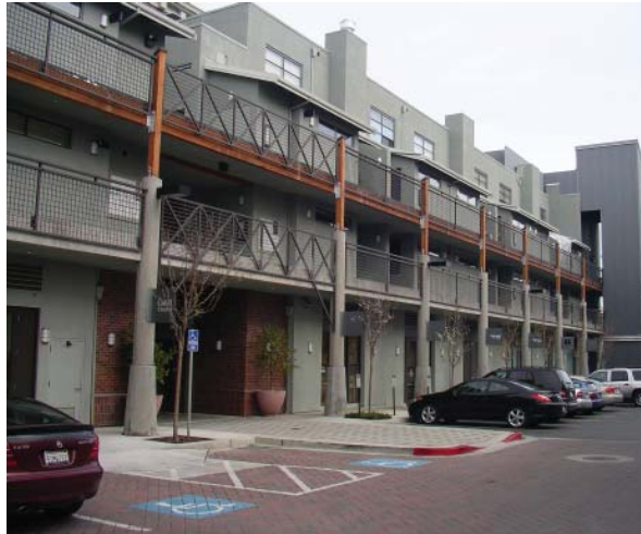
Example of desirable front (top) and back building facades of high intensity mixed-use TOD building
