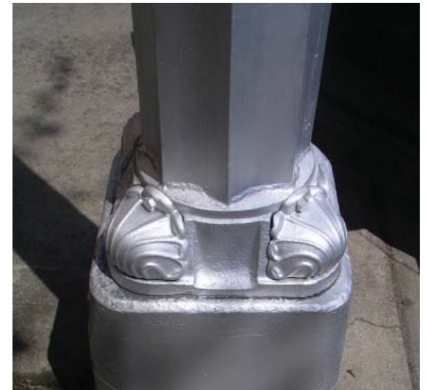
Unique street lights at Globe and Arden/Del Paso Stations
