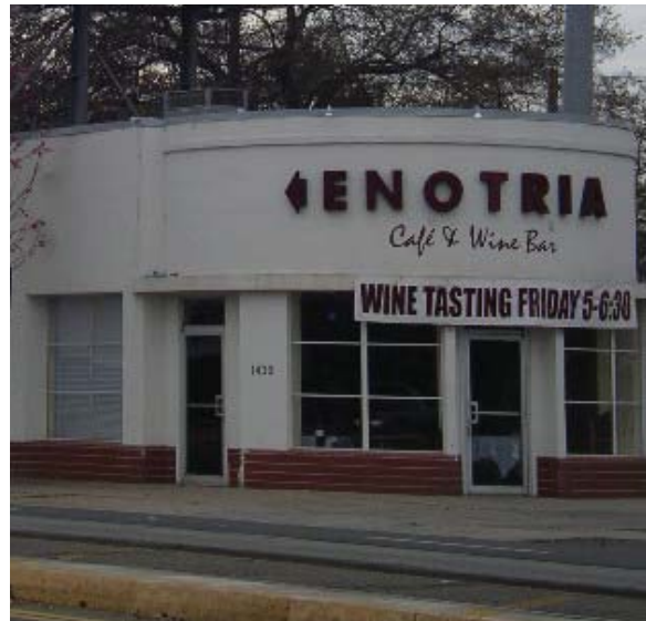
Character-defining buildings at the Arden/Del Paso Station
