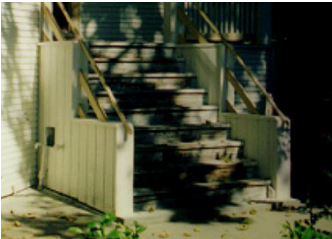
Figure 3-56. 614 25th Street. Inappropriately used exterior materials, and lack of detailing, can lower the quality and value of properties.
