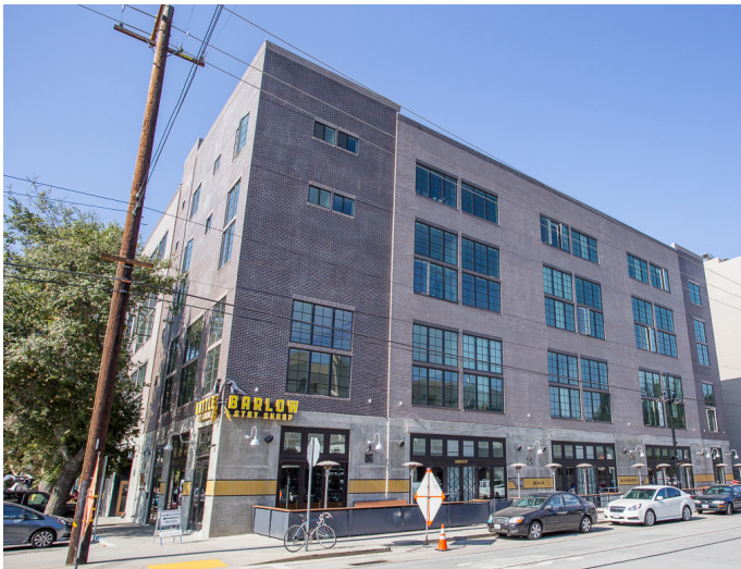
Figure 3-46. Appropriate window treatment can be achieved by providing smaller individual windows or by staggering wall planes.
