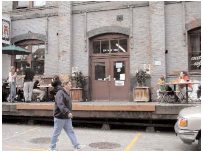
Figure 6-39. Sections of the historic Pearl neighborhood in Portland typify a shared public realm and provide a model for potential development along R Street.
