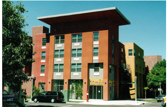
Figure 3-37. 17th and K Streets. A large variety of materials and forms are carefully studied to provide a cohesive theme.
