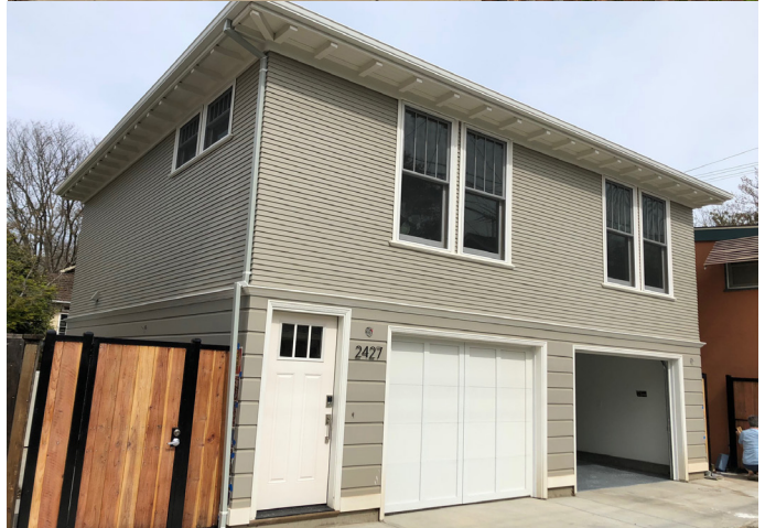
Figure 3-81 and Figure 3-82 : Enhancement of a residential alley by the construction of infill structures on single lots.
