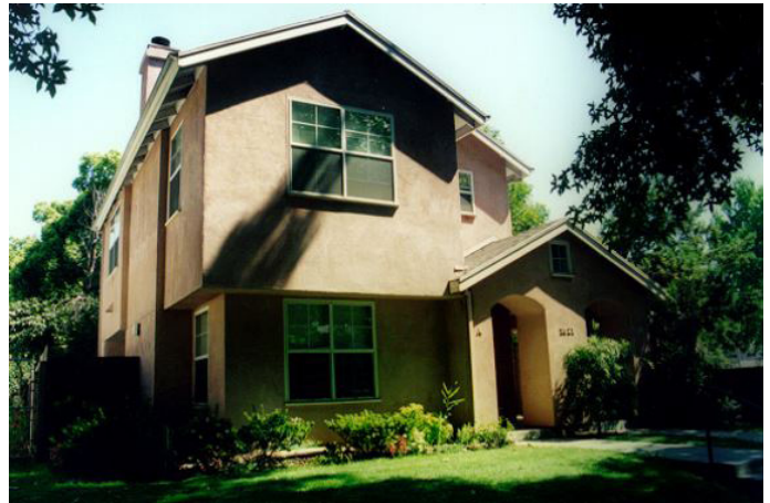
Figure 3-58. 1521 V Street. When plaster is used, smooth plaster texture is most compatible in the Central City.
