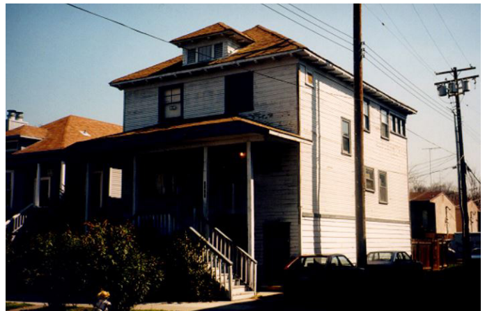
Figure 3-71. 1715 23rd Street. The modifications to the porch are inconsistent with the original character of the house.
