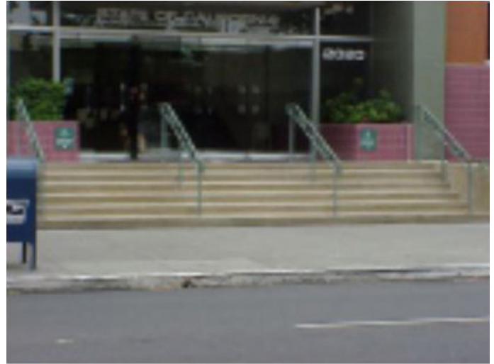
Figure 3.57. State EPA Building, L Street
