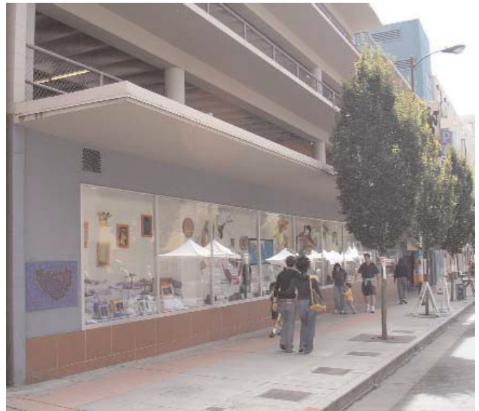
Figure 6-52. As seen in a downtown Berkeley parking structure, blank walls, such as those in Sector C, can be transformed into public gallery space to create an engaging pedestrian experience.
