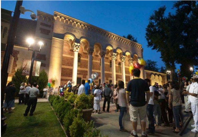
Figure 3-59. Outdoor lighting is used to enhance the architectural features of the Sacramento Memorial Auditorium.
