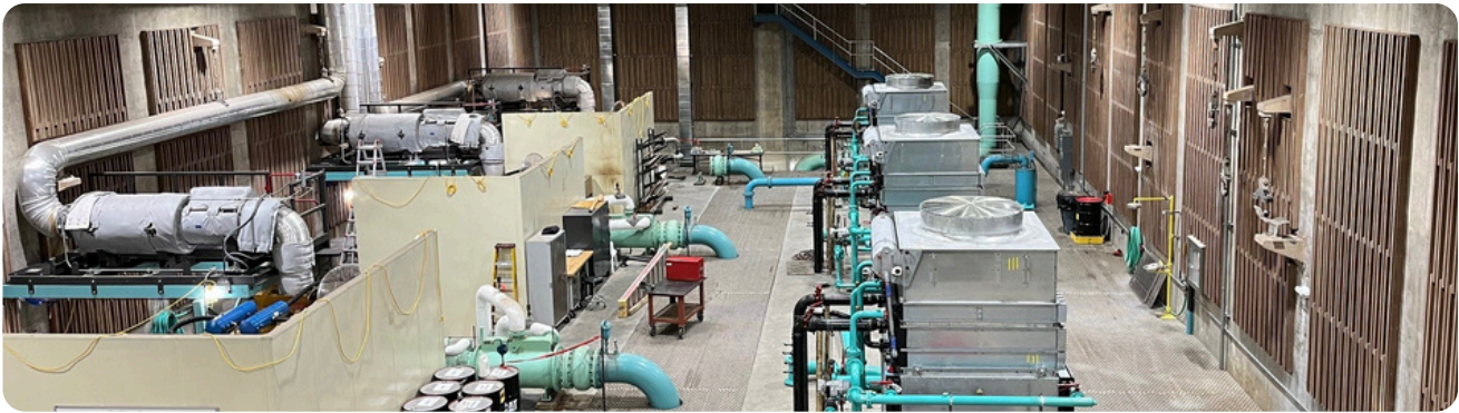
Florin Reservoir after LED lighting retrofit
