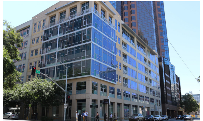
Figure 2-13. The building facade 800 J Street re-interprets traditional rhythm of street wall by suggesting different building widths and fenestration
