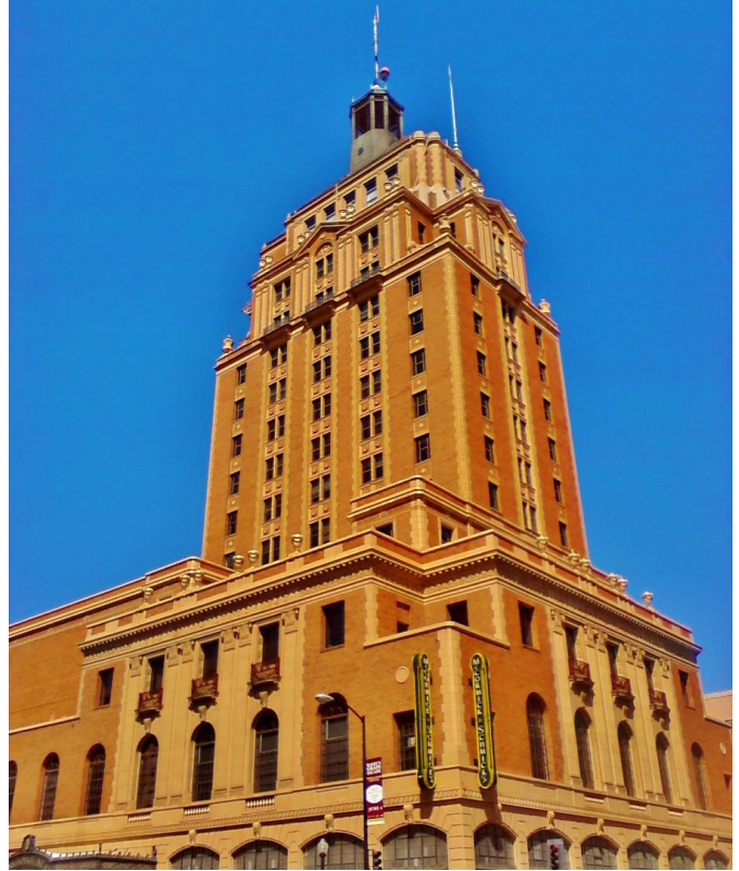
Figure 2-18. Elks Building - The integration of brick with terracotta accents highlight the stepped massing and slender tower of this early 20th Century landmark.
