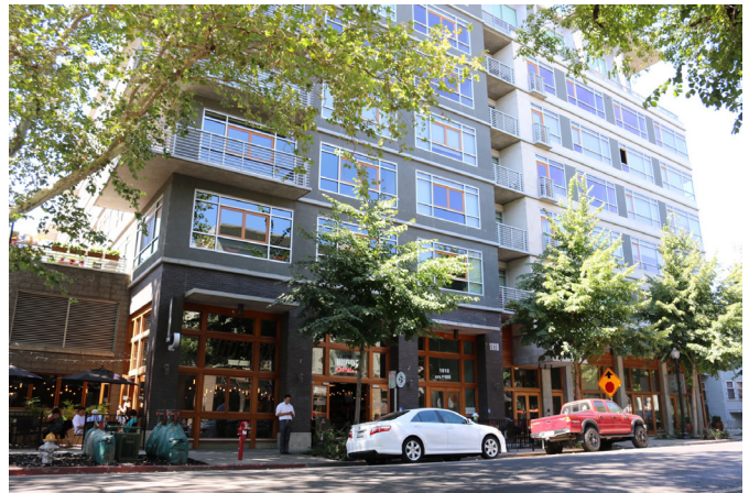
Figure 2-3. The L Street Lofts in Midtown demonstrate well-designed neighborhood retail integrated into the ground floor.
