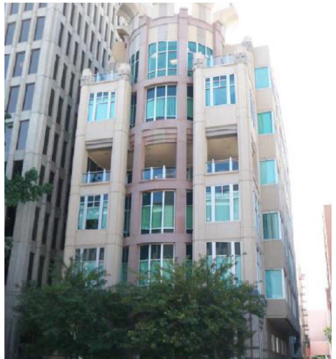
Figure 2-15. An Infill Project exemplifying the 40-foot rhythm of Sacramento's historic block platting and subsequent building facades.
