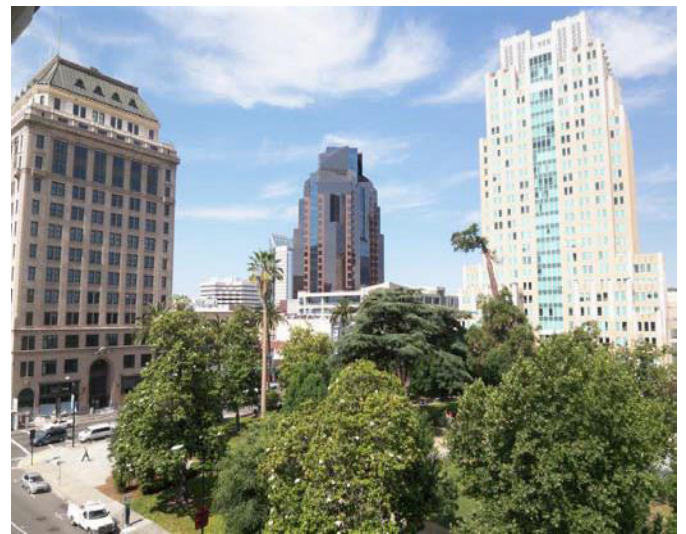
Figure 2-6. Building on left represents traditional historic form with vertical ribbons of punched window groupings, strong base, middle and a distinctive roof top. The street wall is well defined with a hierarchy of horizontal comicing utilizing local terracotta exterior details and cladding. High rise tower in center exhibits “contrasting” architectural elements to interject visual tension to skyline. High-rise tower at right side employs creative re-interpretation of “punched” fenestration groupings. The building massing, distinctive roof top element and exterior coloration harmonize with the neighboring historic structures.
