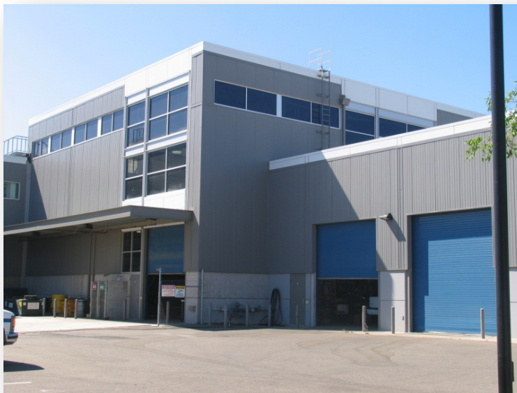
Image 2.12: Loading area integrated into the design of project with no equipment being visible on the outside of the structure
