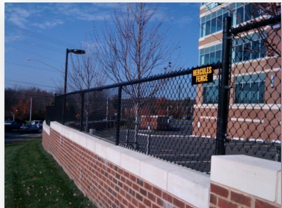
Image 1.8: Vinyl coated chain-link fencing is encouraged over galvanized chain-link or wood fence material
