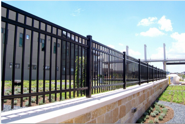
Image 1.7: Wrought iron fencing, combined with landscaping and materials compatible with the development
