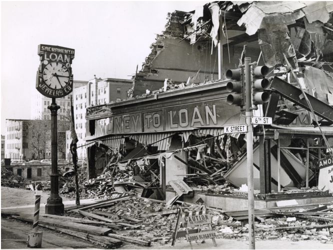
View of the demolition in the West End of the buildings at 531 K Street to make room for the new K Street Mall project.
