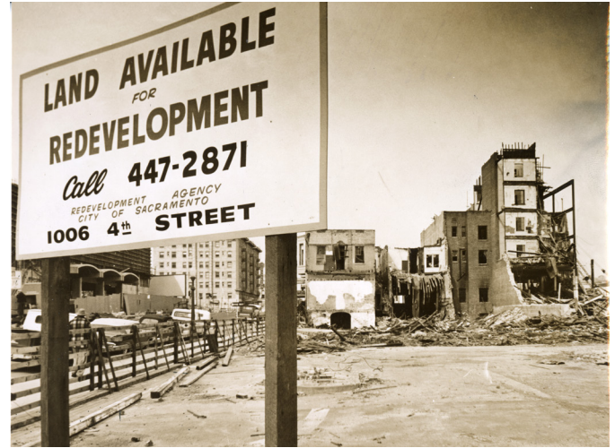
“Land Available for Redevelopment” by the City of Sacramento’s Redevelopment Agency and the West End project. View is looking north toward K Street from 5th and L Streets.
