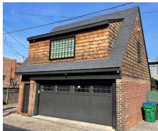
FIGURE 11: EXAMPLE OF PANELED GARAGE DOOR WITH VIEWING WINDOWS. WINDOWS MAY BE FAUX OR ONE-WAY VIEWING WINDOWS.
