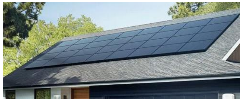
FIGURE 13: SOLAR PANELS SHALL BE MOUNTED PARALLEL WITH THE ROOF.
