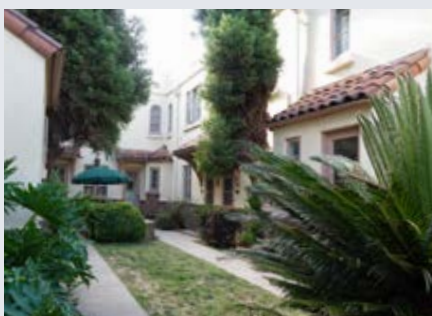
Courtyard Building Central City
