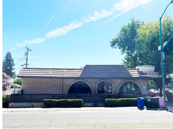
Figure 2. Northeast facade, view southeast.
