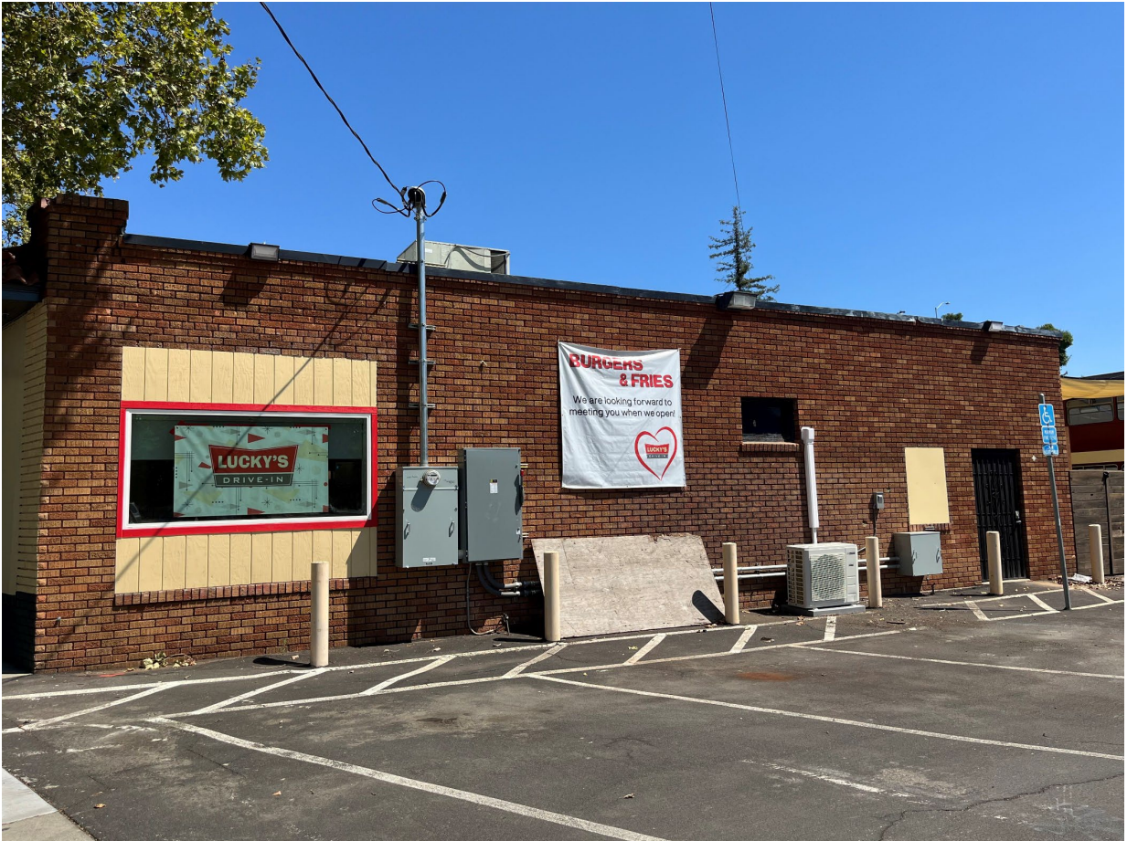
Figure 1. South facade, view northeast.
