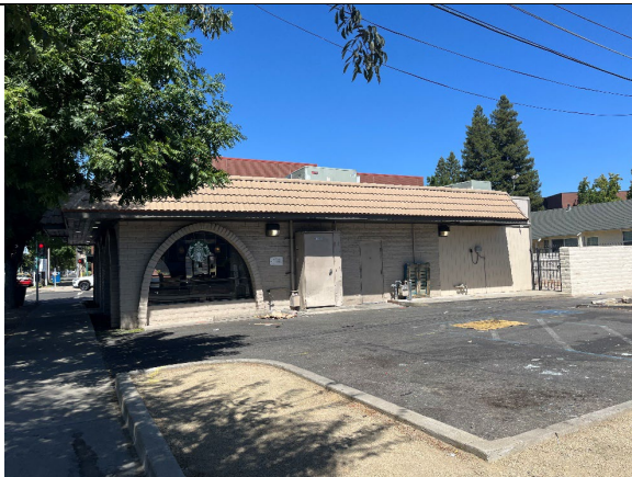
Figure 3. Southwest facade, view north.
