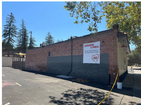
Figure 3. North facade, view southeast.
