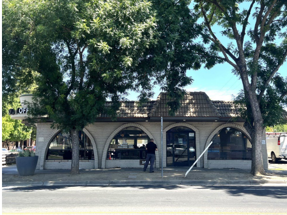
Figure 1. Northwest facade, view southeast.
