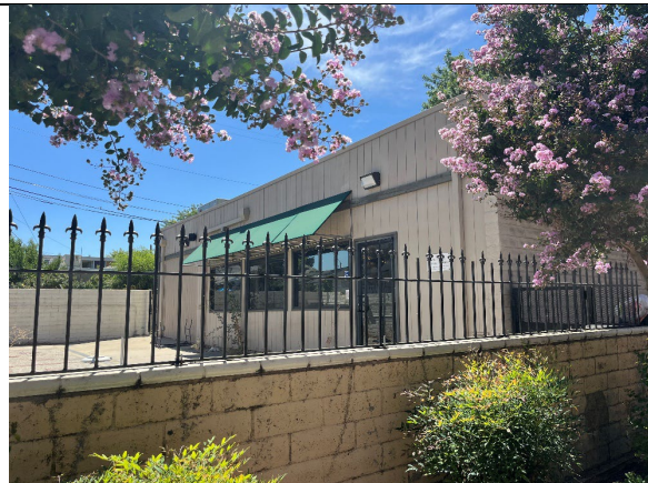
Figure 4. Southeast facade, view west.
