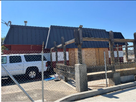
Figure 1. North facade, view southwest.
