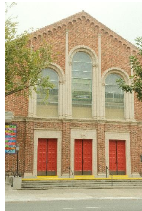
FIGURE 12: 2100 J STREET'S CHARACTER-DEFINING FEATURES INCLUDE LARGE CARVED WOOD DOORS AND STAINED-GLASS WINDOWS.
