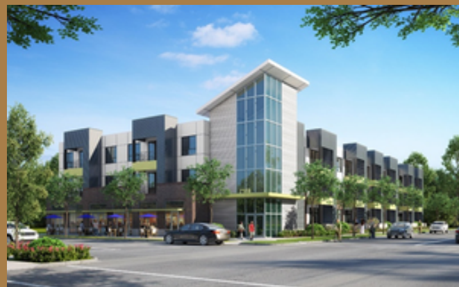
3rd and S Street Mixed-Use Building
