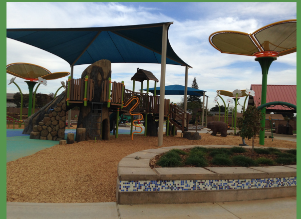
Artivo Guerrero Park - Formerly a dilapidated private swim club, the property was redeveloped as a neighborhood park with several pools and a clubhouse. The park was developed with a $2.8 million Proposition 84 grant and reopened in November 2014.
