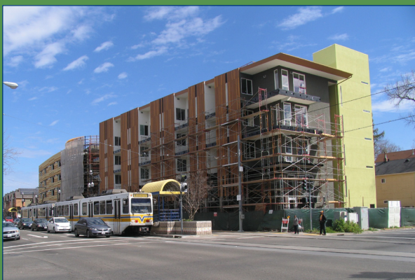
La Valentina - 12th and E Streets Under Construction
