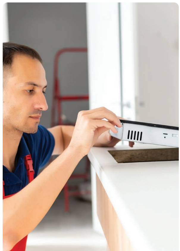
Induction Stove Installation
