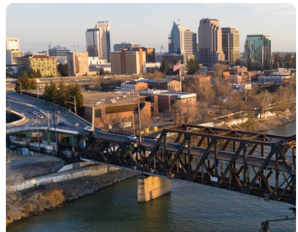
I Street Bridge and Downtown Sacramento
