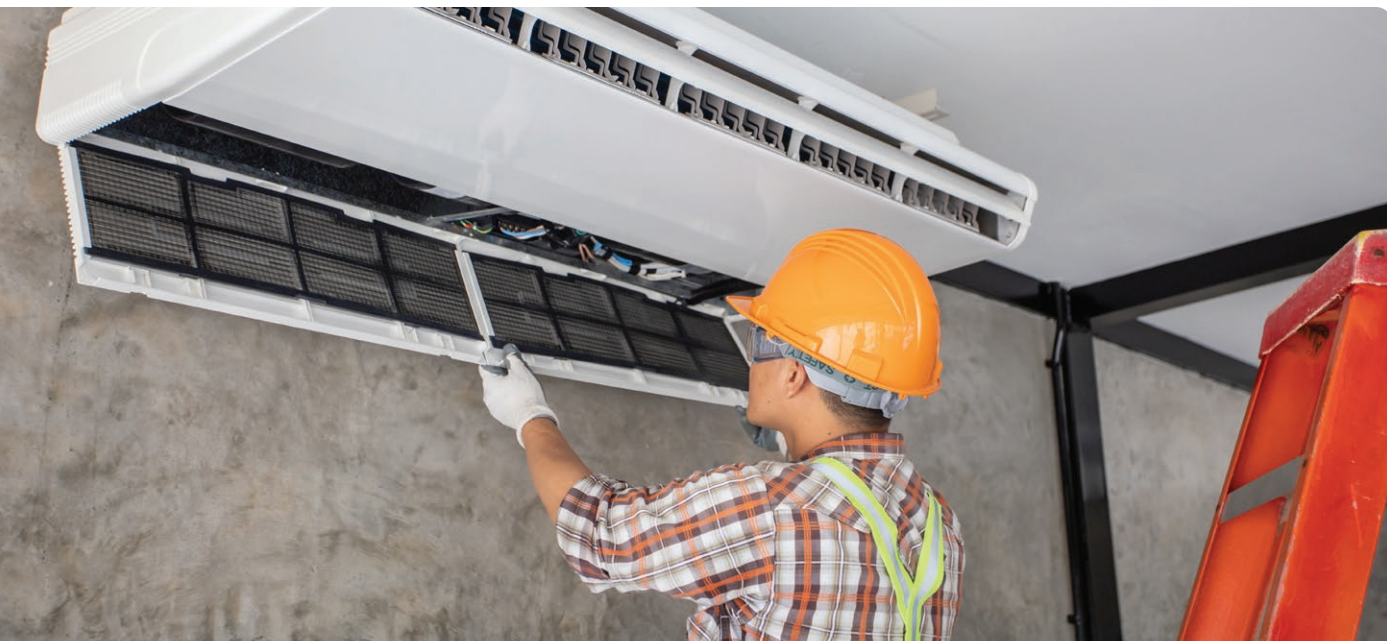
Electric Heat Pump HVAC Unit Installation
