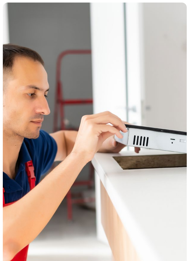
Induction Stove Installation
