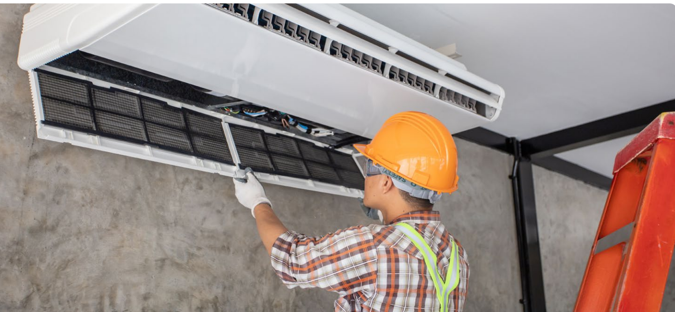
Electric Heat Pump HVAC Unit Installation
