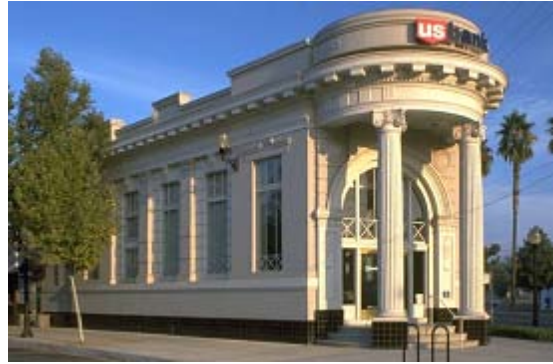
The US Bank Building in Oak Park, Sacramento's first suburb
