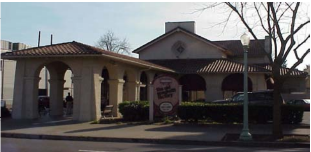
Former Western Pacific Depot at 1910 J St.
