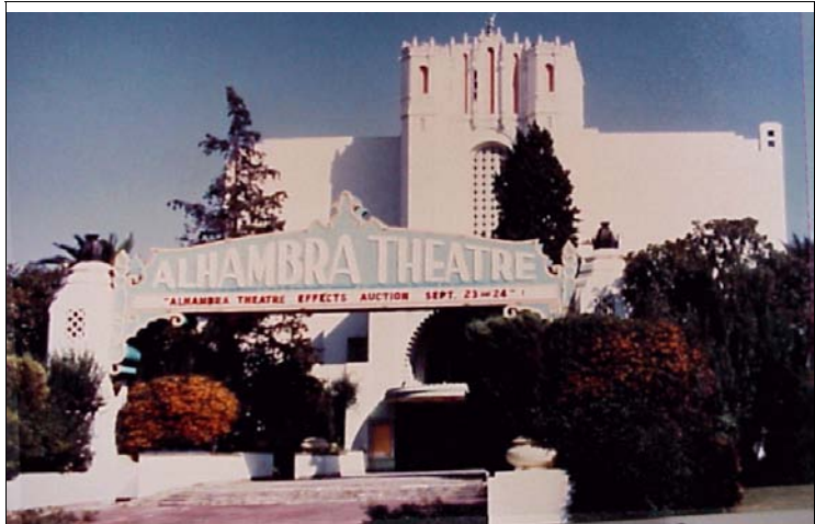
Demolition of the Alhambra Theatre in the 1970s spawned Sacramento’s modern preservation movement
