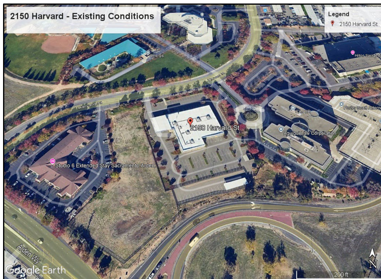
FIGURE 4: PROJECT SITE - EXISTING CONDITIONS
