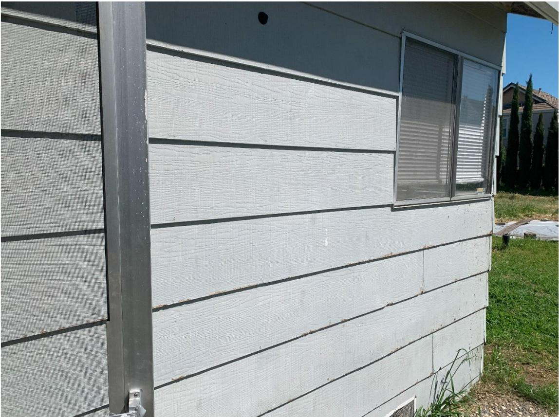
Transite (asbestos) siding typical of that on residence and garage.
