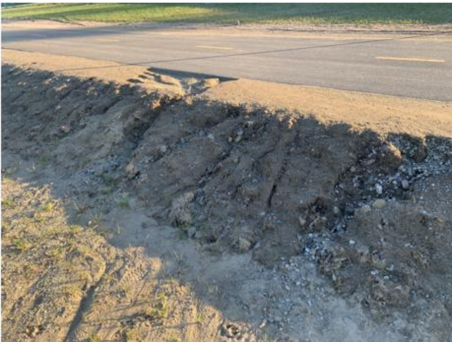
Two Rivers Bike Trail ADA Access Ramp Glenn Hall--AR Parkway
