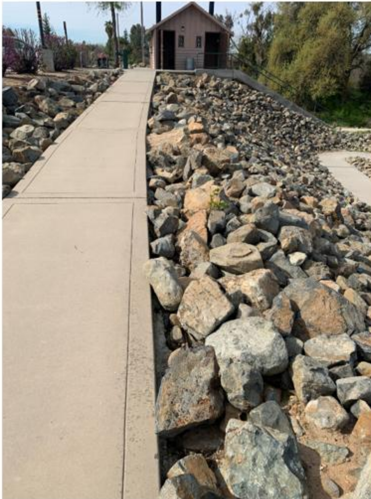
Friant Cove ADA Ramp & Riprap, San Joaquin River Parkway below Friant Dam
