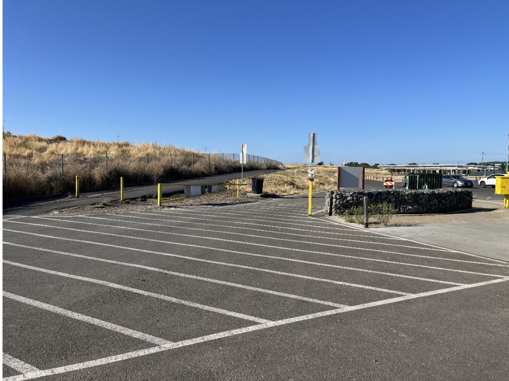
Photo 3. Representative of the urban areas within the BSA featuring a paved parking lot, skate park and trail. Taken facing south (June 2025).
