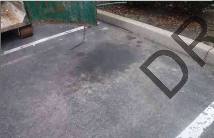
Photo 3: Oil Stains in Parking Lot
