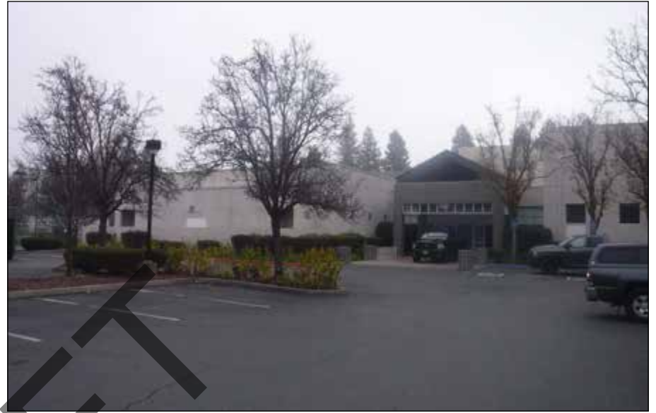
Photo 2: Main Sports Complex Facing Northeast
