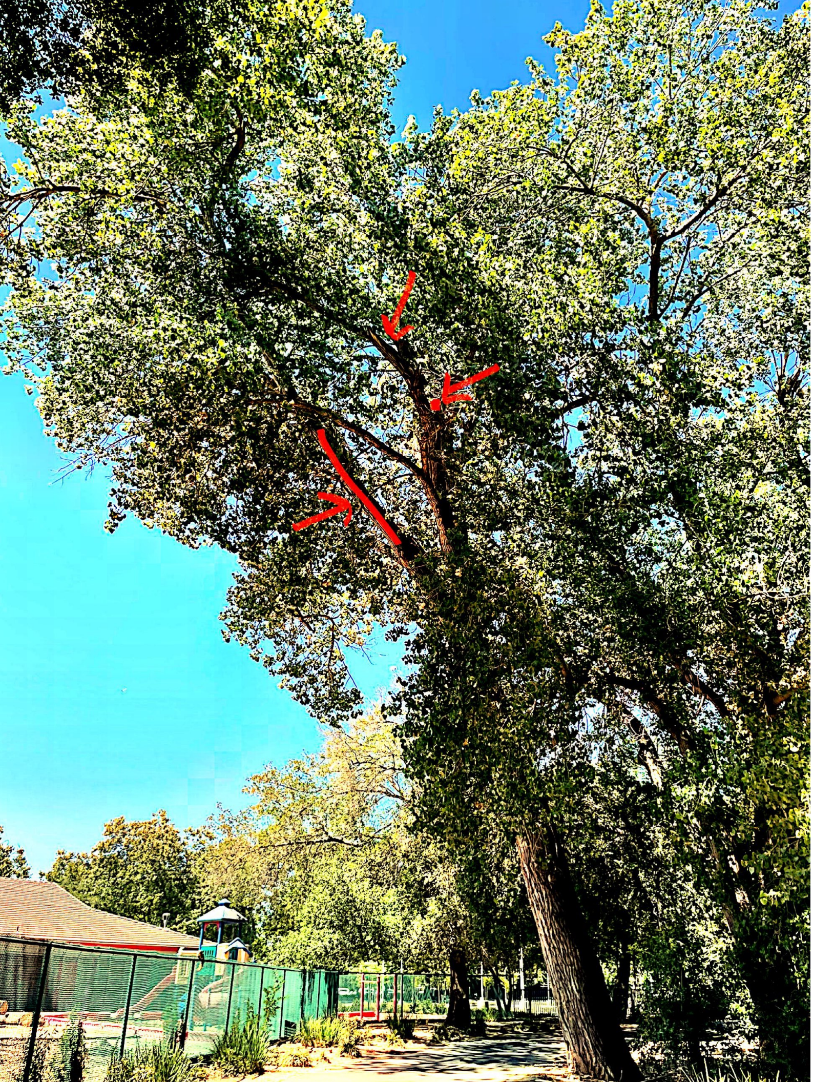
Shows Lean toward schood yard
