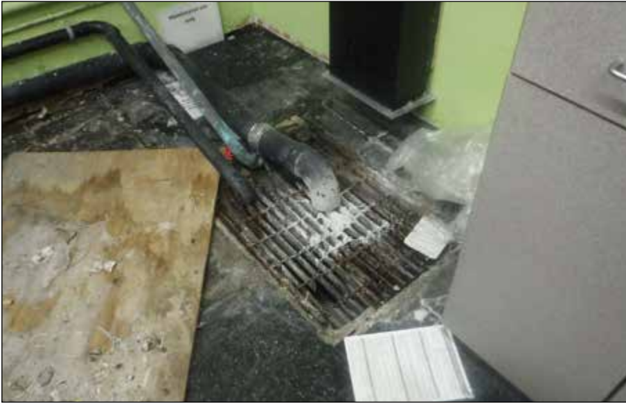
Photo 5: Laundry Room Drain
