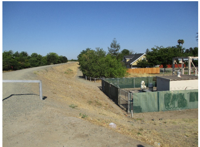
Photo 16. View looking west on the land side of the levee. Sump 103 occurs in the fenced facility on right. 23 July 2020.
