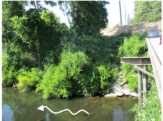
Photo 2. View looking north toward Steelhead Creek. The Sump 58 Outfall Channel is obscured by riparian vegetation at center. 23 July 2020.
