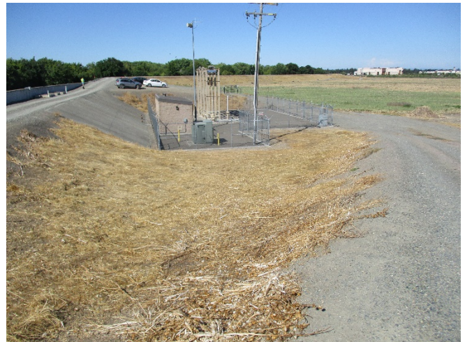
Photo 8. View looking southwest toward the nonnative grassland on the land side of the levee and Sump 89. 22 July 2020.
