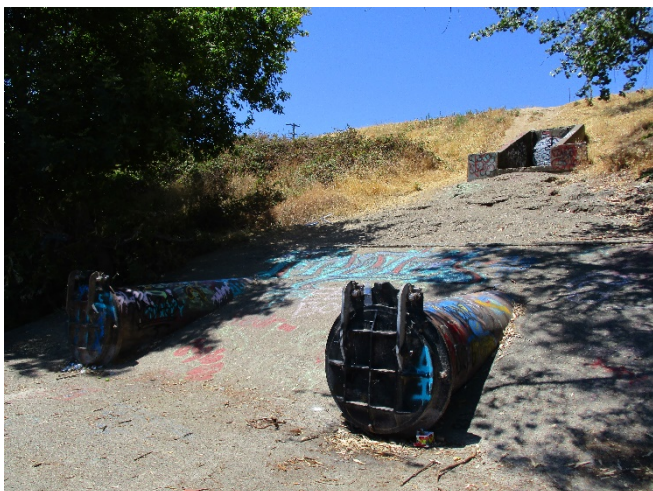
Photo 25. View looking southwest toward the Sump 155 outfall structure. 22 July 2020.
