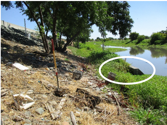
Photo 7. View looking northeast toward the Sump 89 outfall (circled). Data Point 1 is located at shovel in foreground. 22 July 2020.
