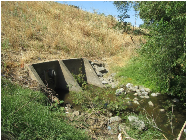
Photo 29. View looking southwest toward the Sump 159 outfall into Arcade Creek. 23 July 2020.
