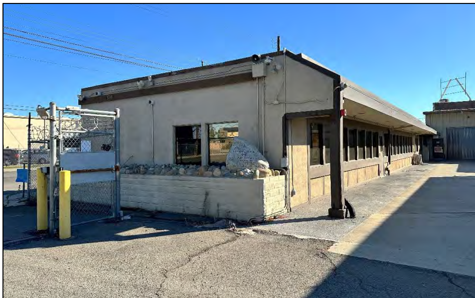
Photograph 2: Office building, camera facing northeast, November 10, 2022.
