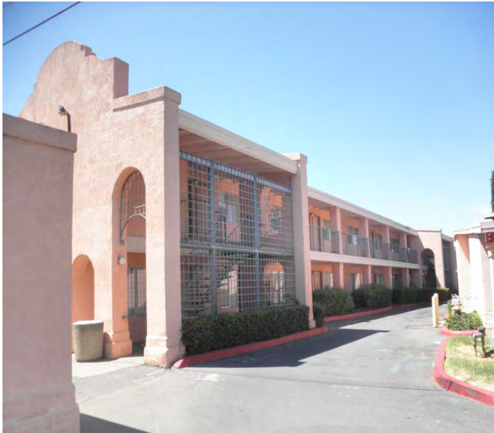
Building 700; facing northwest. July 17, 2015
