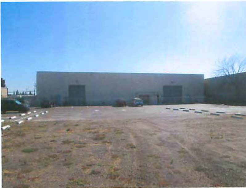
Photo 8: Looking east at the back side of the structure
