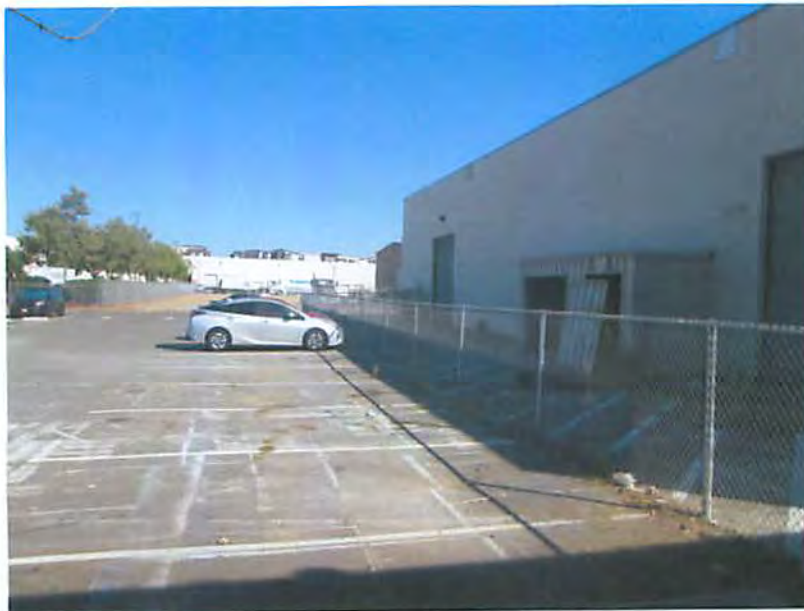
Photo 10: Looking north at the back side of the structure
