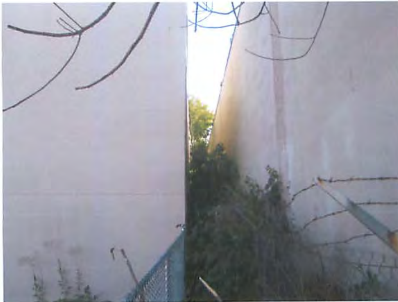
Photo 12: Looking east at the side of the structure
