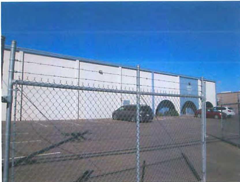
Photo 2: Looking northwest at the Subject Property
