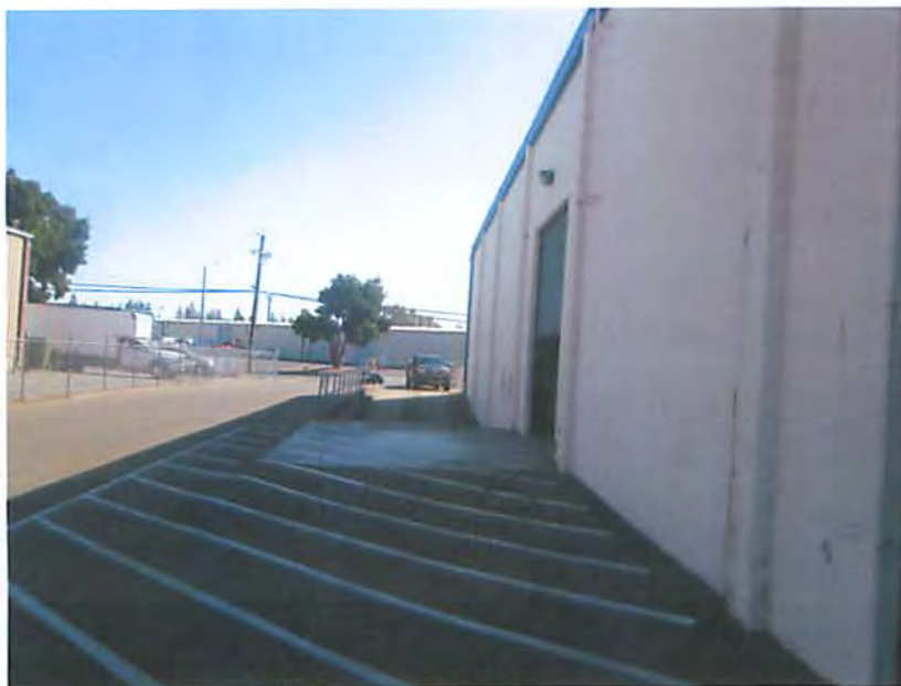
Photo 6: Looking east at the side of the warehouse
