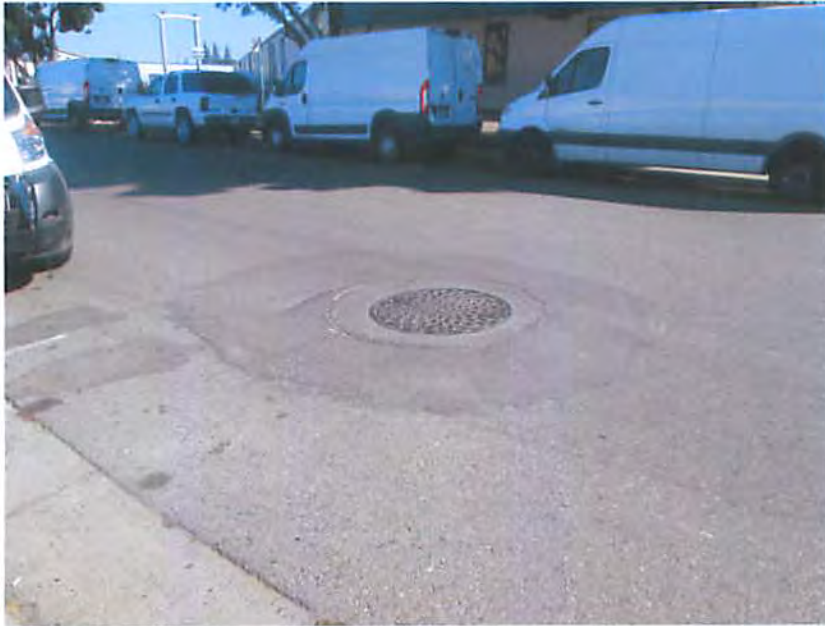
Photo 1: Looking at the Sewer connection on Ramona Avenue
