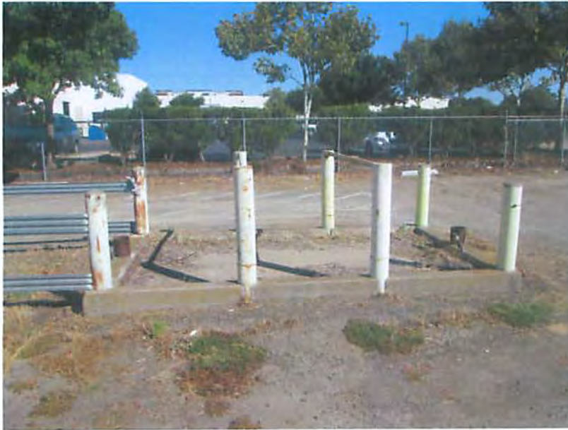
Photo 9: Looking at former area for potentially holding hazardous materials
