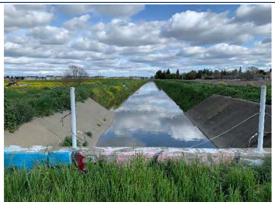
Easterly view from westerly portion of onsite drainage canal
