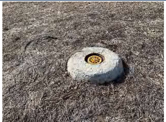
Apparent sewer pipe access port/clean-out on far easterly margin of the property
