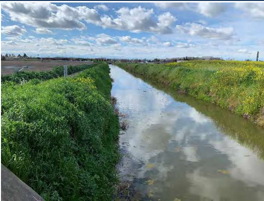
Westerly view from easterly portion of onsite drainage canal
