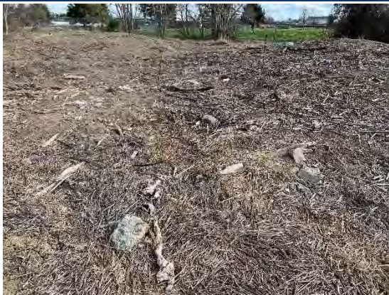
Apparent fill piles containing concrete rubble and debris along southerly margin of the property
