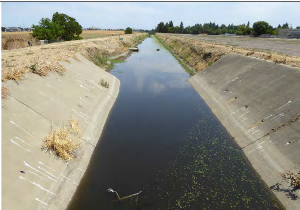
2. Canal looking east from the west end
