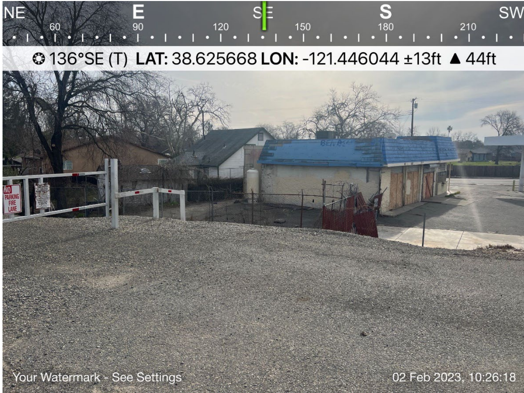
Photo 3: Project site from the northern end facing SE
