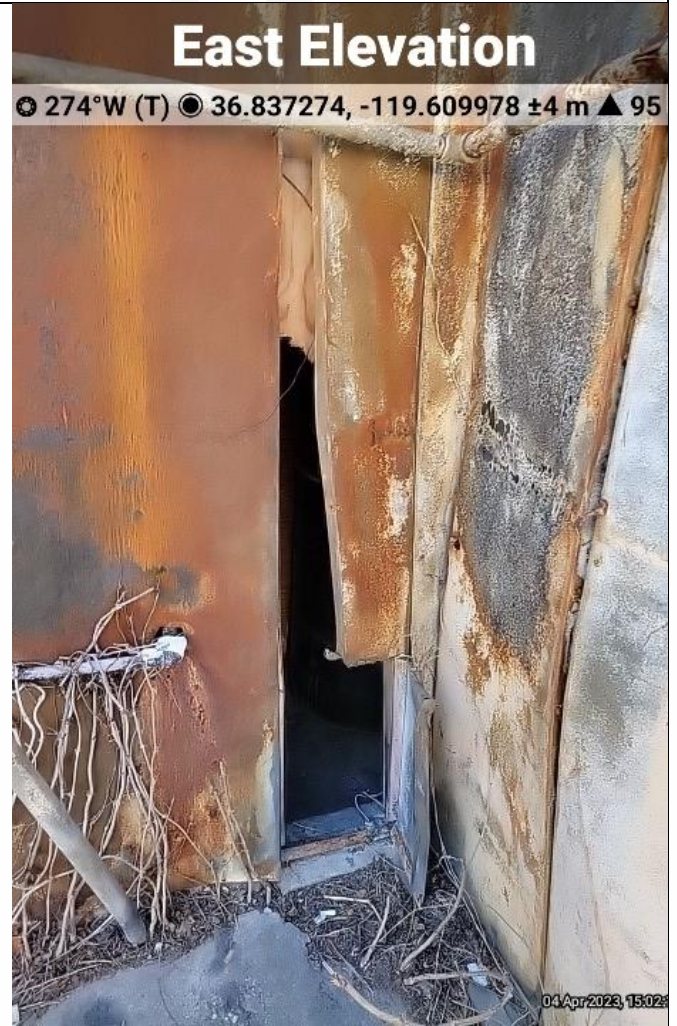
Photo 16 – East corner of the site (Facing West).
