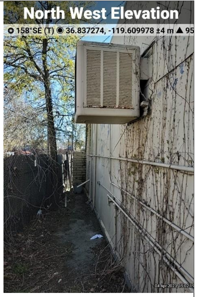
Photo 28 – Evaporative cooler present on rear of building. View southeast.
