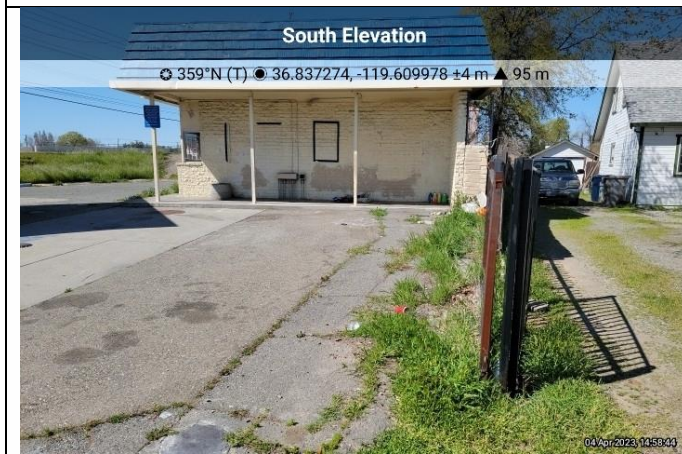
Photo 9 – South corner of the site (Facing North).
