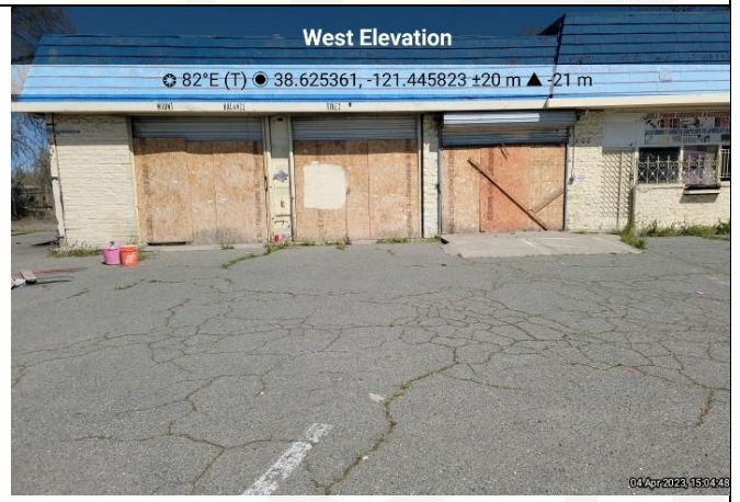
Photo 6 – West corner of the site (Facing East).
