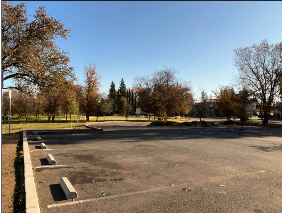
Photo D-7. View looking east at parking lot near southeast corner of BSA.
