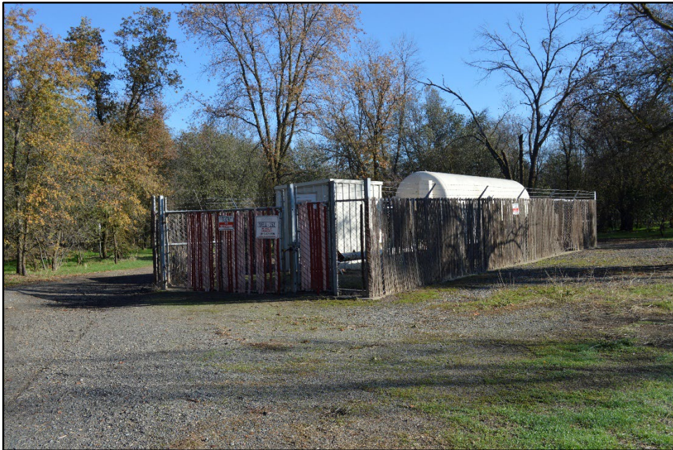
Figure 13. Pumphouse and aboveground storage tank at the northeast corner of the property, view east.
