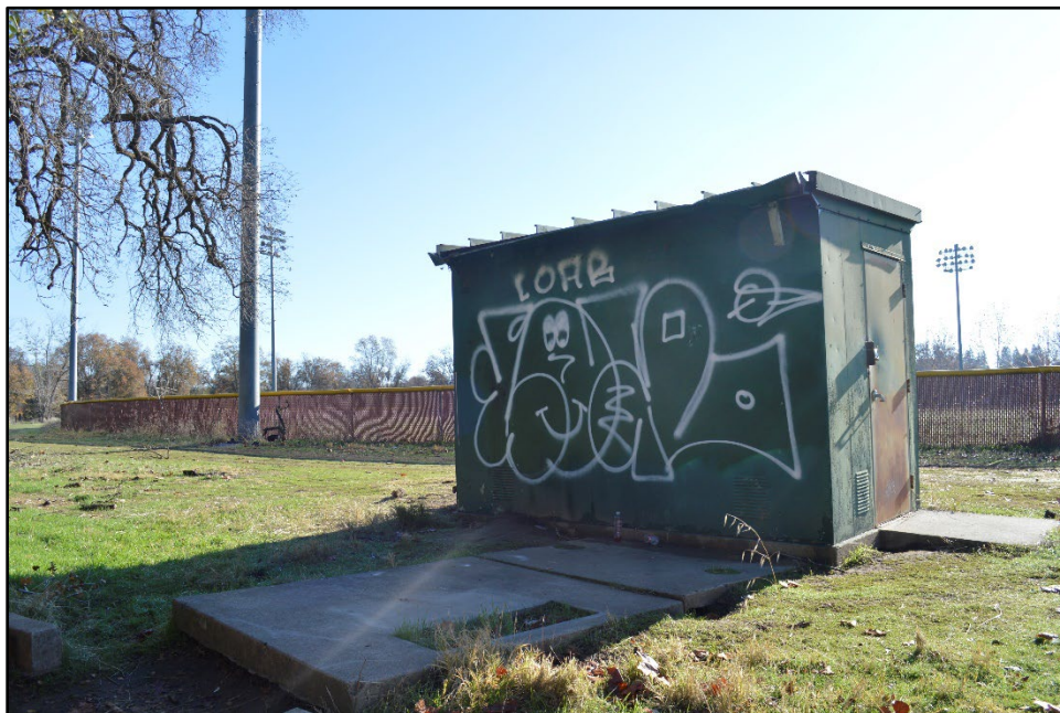
Figure 9. Utility Shed located north of Renfree Field, view southeast.
