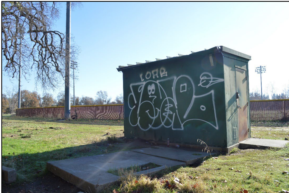
Figure 44. Utility Shed located north of Renfree Field, view southeast.
