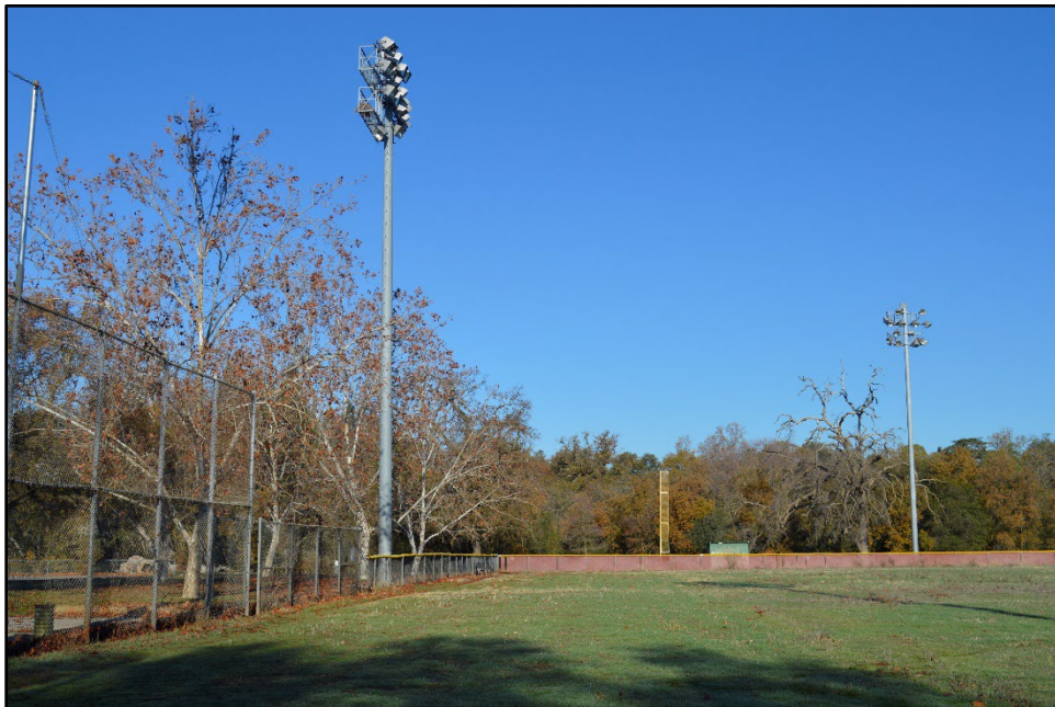
Figure 39. Typical chain-link fencing, lighting, and foul ball post at Renfree Field's left field, view north.
