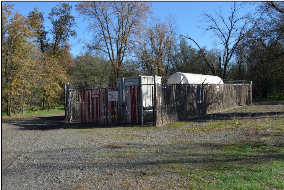
Figure 13. Pumphouse and aboveground storage tank at the northeast corner of the property, view east.
