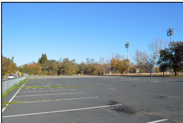
Figure 27. Overview of the surface parking lot, view north.
